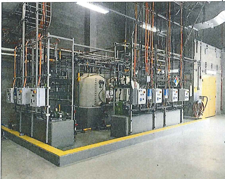
Photo # 23 Image: IMG_0284 Date: 6/25/2019 Taken by: Amy Jankowiak Description: Sodium hypochlorite dosing pumps and chemical day tanks (background). Pumps supply hypochlorite to C3 water system, both reclaimed water systems, and effluent disinfection system.
