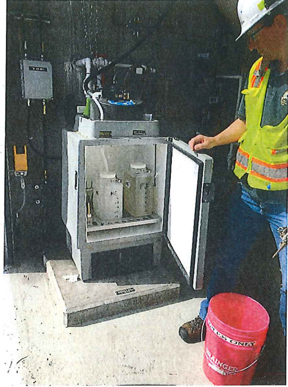
Photo # 34 Image: IMG_0124 Date: 6/25/2019 Taken by: Shawn McKone Description: Membrane effluent composite sampler at MEB.
