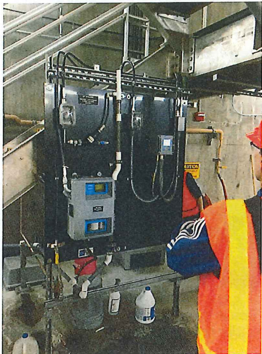
Photo # 5 Image: IMG_0110 Date: 6/25/2019 Taken by: Shawn McKone Description: Effluent continuous chlorine monitoring at IPS
