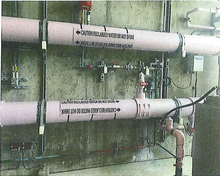
Photo # 25 Image: IMG_0281 Date: 6/25/2019 Taken by: Amy Jankowiak Description: Disinfection contact pipe network for reclaimed water distribution system.
