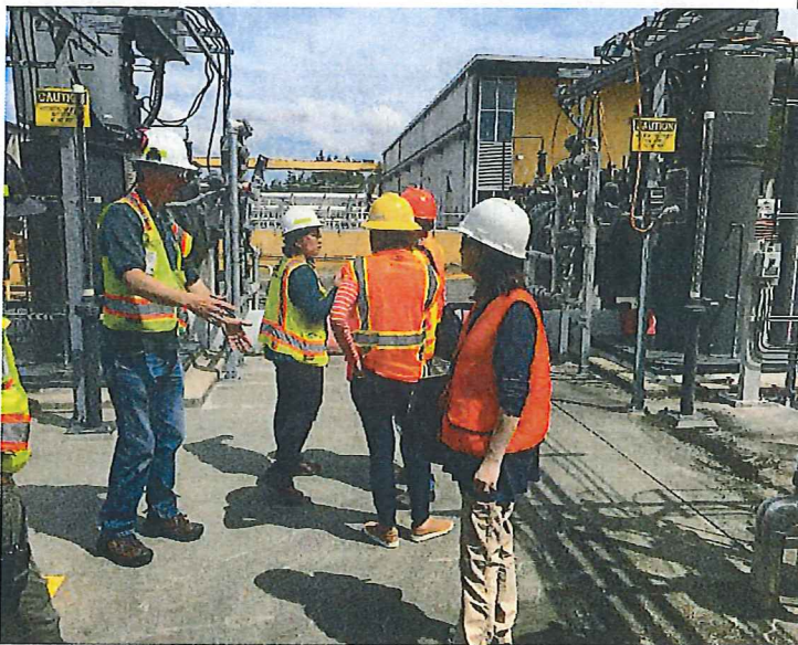
Photo # 19 Image: IMG_0166 Date: 6/25/2019 Taken by: Shawn McKone Description: Mixed liquor feed pumps (behind group) from aeration basins to membrane basins.
