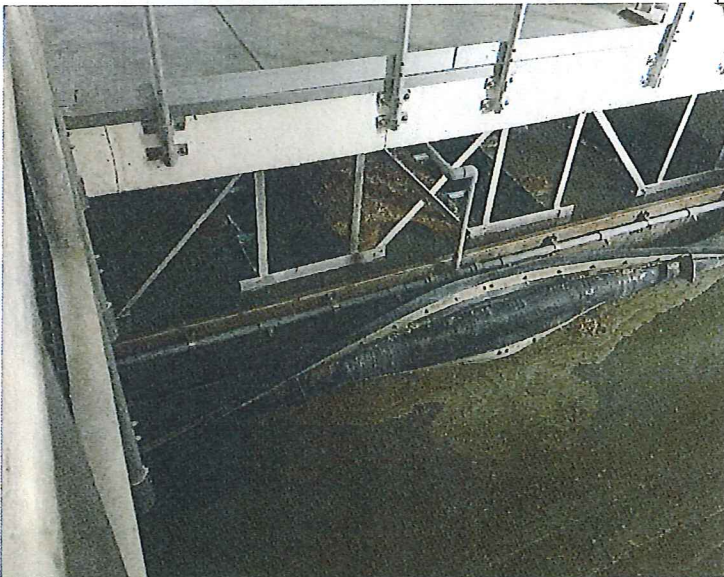
Photo # 15 Image: IMG_0156 Date: 6/25/2019 Taken by: Shawn McKone Description: Scum skimmer and effluent launders in primary clarifier.
