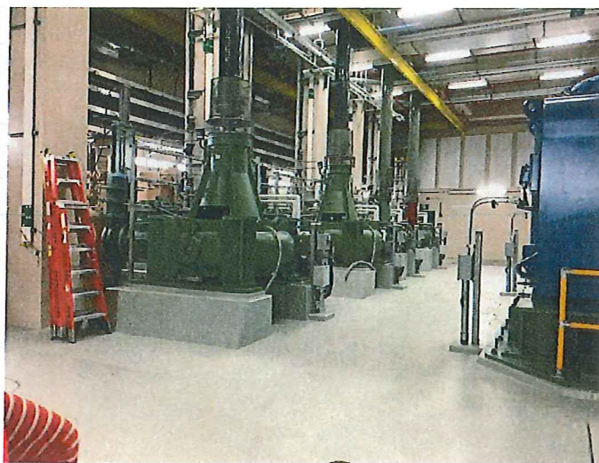
Photo # 10 Image: IMG_0104 Date: 6/25/2019 Taken by: Shawn McKone Description: Raw sewage pumps at IPS.
