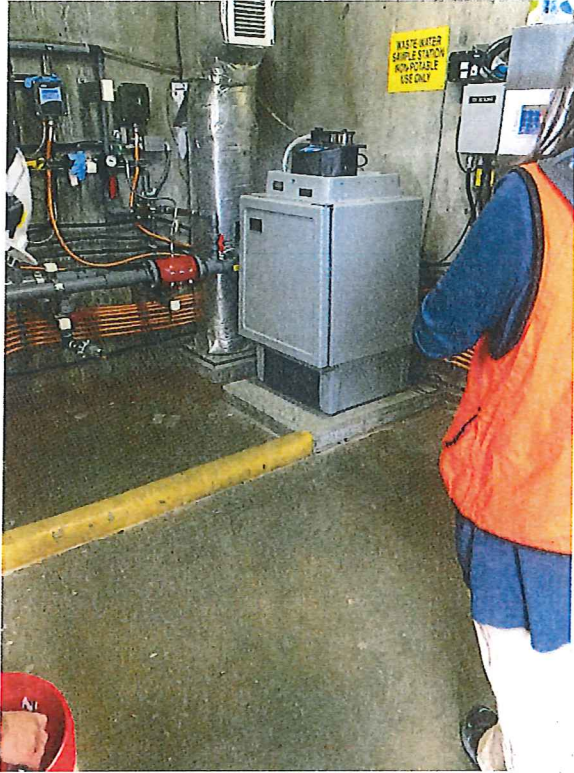
Photo # 33 Image: IMG_0133 Date: 6/25/2019 Taken by: Shawn McKone Description: Influent composite sampler at headworks.
