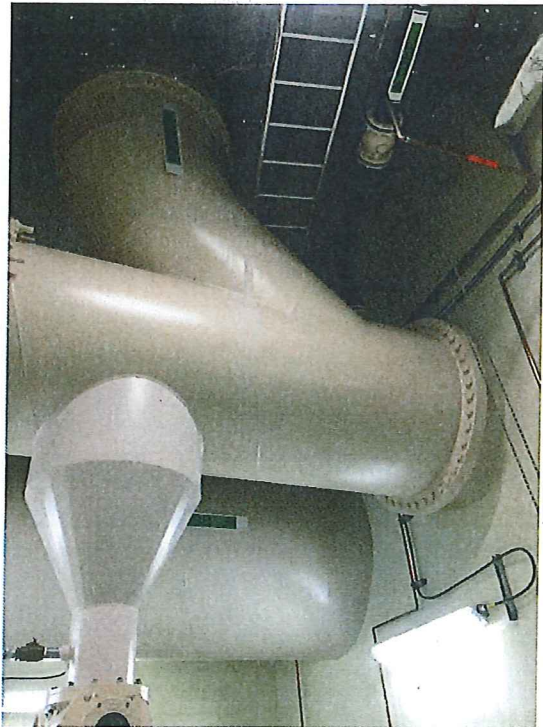
Photo # 11 Image: IMG_0149 Date: 6/25/2019 Taken by: Shawn McKone Description: Raw sewage influent force mains at Brightwater facility – distribution channel to screens located one level above.
