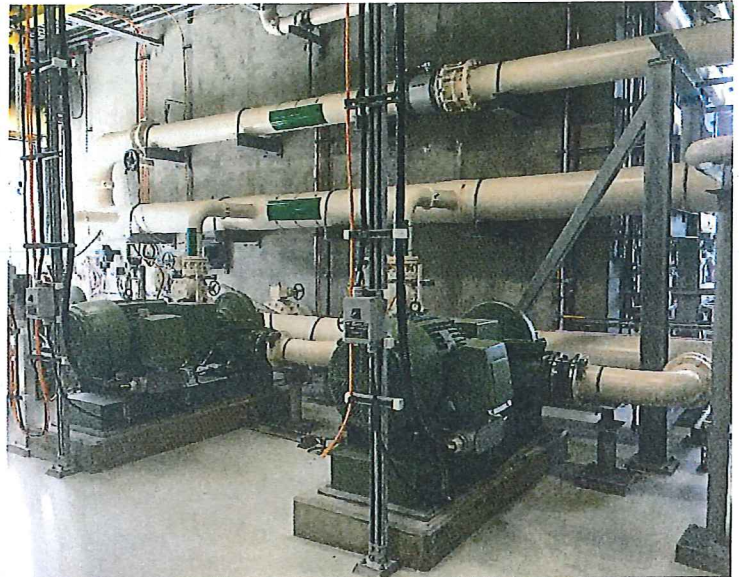
Photo # 22 Image: IMG_0132 Date: 6/25/2019 Taken by: Shawn McKone Description: High-pressure "C3" utility water pumps inside disinfection building. Wall to MEB is behind the pumps, supporting the C3 water pipes.
