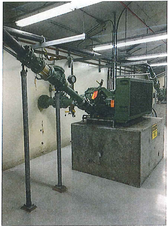
Photo # 14 Image: IMG_0152 Date: 6/25/2019 Taken by: Shawn McKone Description: Grit classifier pump located below the grit basins.
