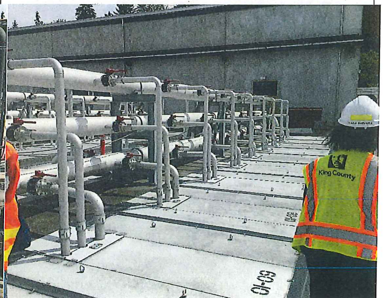
Photo # 20 Image: IMG_0168 Date: 6/25/2019 Taken by: Shawn McKone Description: Process air (top 2 lines) and membrane effluent suction (bottom line) headers for membrane basin 3.
