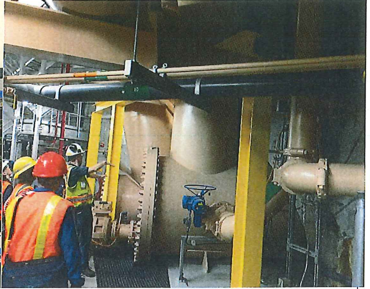
Photo # 2 Image: IMG_0107 Date: 6/25/2019 Taken by: Shawn McKone Description: Raw sewage force mains to Brightwater facility at IPS.
