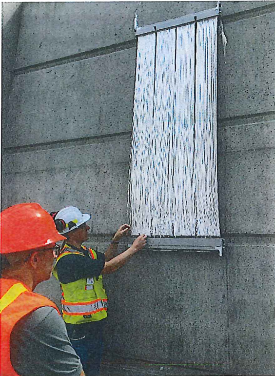
Photo # 21 Image: IMG_0169 Date: 6/25/2019 Taken by: Shawn McKone Description: Sample membrane module displayed outside of the membrane basins.
