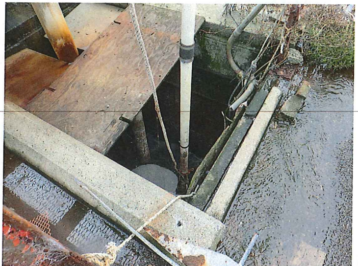
PHOTO #2: WET WELL FOR WASTEWATER HOLDING FROM FISH PROCESSING AREAS. SEAWATER OVER FLOW SHOWN FROM CRAB WASHING
