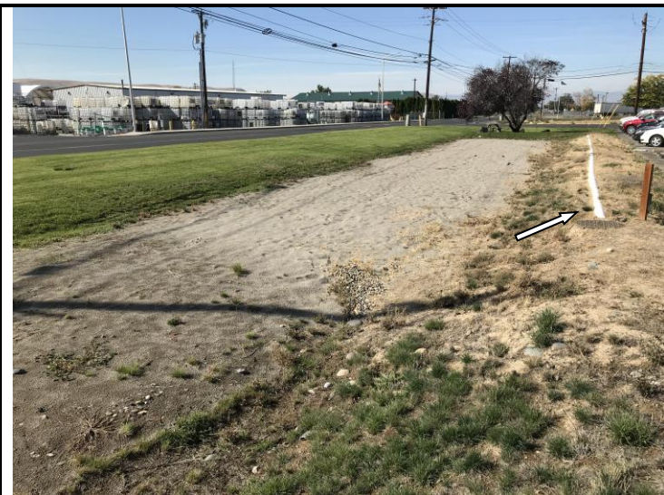
FIGURE 1: INFILTRATION SWALE TO SOUTH HAS PUMP AND AN EXPOSED PERFORATED PIPE.
