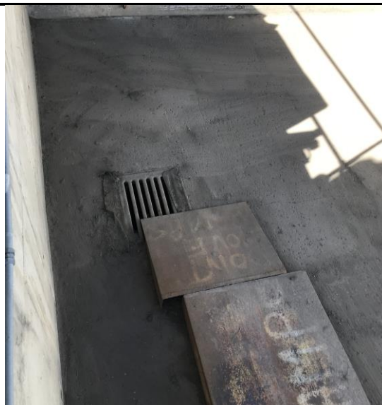
FIGURE 2: EAST LOADING DOCK CATCHBASIN HAS INSERT CLOTH AND DRAINS TO BIO SWALE.
