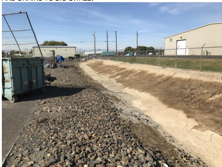
FIGURE 4: INFILTRATION SWALE TO THE NORTH HAS EROSION FROM NEIGHBORS ON-FLOW IRRIGATION
