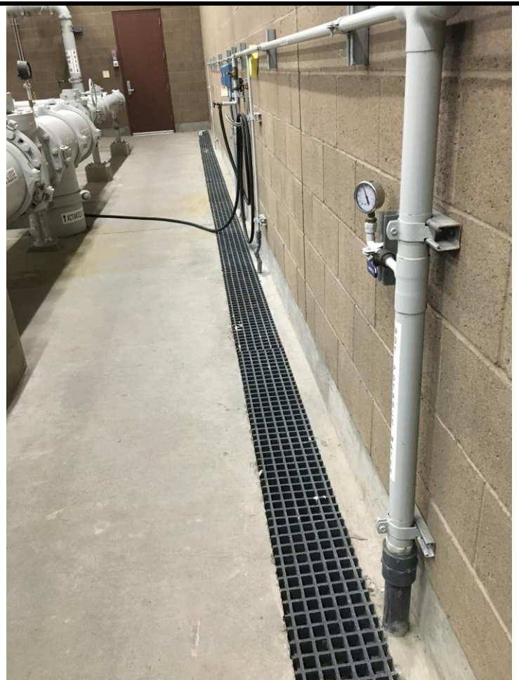
Inside drains connect to water treatment line
