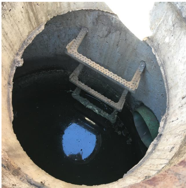
One of 2 drywells, with a tributary storm drain pipe
