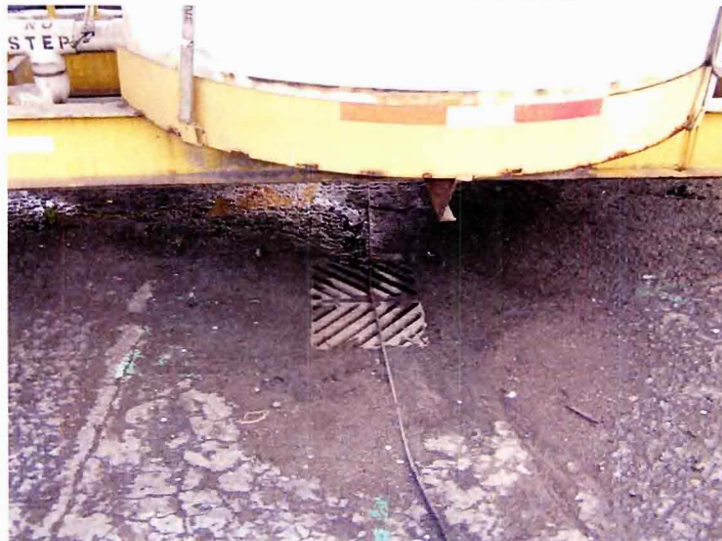
PC050053.JPG DESCRIPTION: STORM DRAIN, LOCATED UNDER PREASURE WASHING TRAILER, RECEIVING PROCESS WASTEWATER FROM LEAK. THICK SEDIMENTATION DEPOSITION HAS ACCUMULATED AROUND THE STORM DRAIN.
