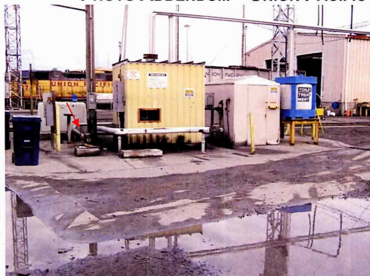
PC050072.JPG DESCRIPTION: OILY RESIDUE FROM FUELING OPERATIONS COAT THE BASE OF THE FUEL PUMP BUILDINGS AND THE PAD OF CEMENT. A LEAKING PIPE DRIPS RED LIQUID ONTO A SATURATED ABSORBANT CLOTH. OIL SHEENS SEEN THROUGHOUT THE PUDDLE.
