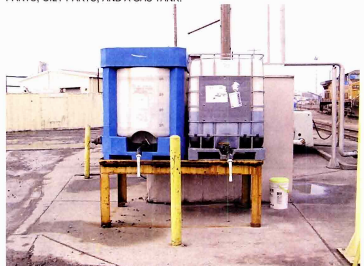
PC050067.JPG DESCRIPTION: CHEMICAL STORAGE WITHOUT SECONDARY CONTAINMENT OR PORPER CHEMICAL HANDLING BMPs IN PLACE (DRIP PANS).
