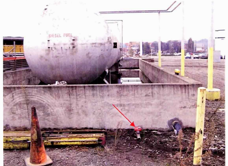
PC050053.JPG DESCRIPTION: EVIDENCE OF DISCHARGE FROM DIESEL TANK CONTAINMENT INTO GRAVEL LOT.
