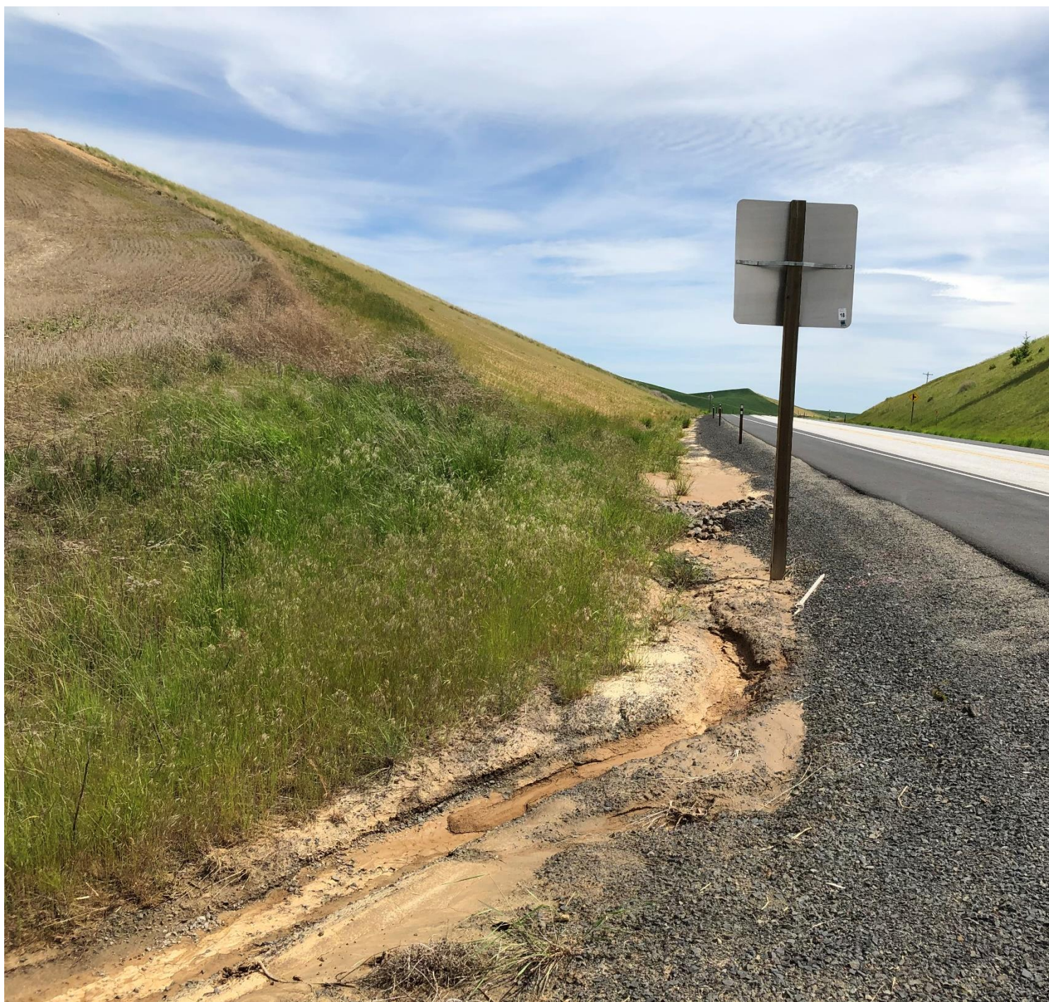
Figure 04 Description: Ditch line below sparse vegetation and rills. Sediment discharging off site towards surface waters.
