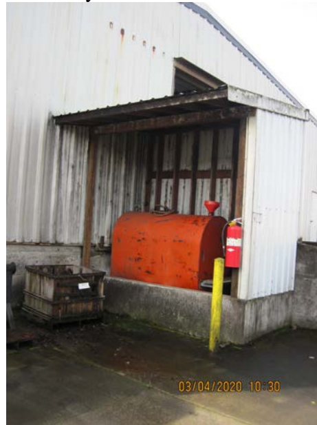
Photo 6 of 6: Their fueling area is covered with secondary containment.
