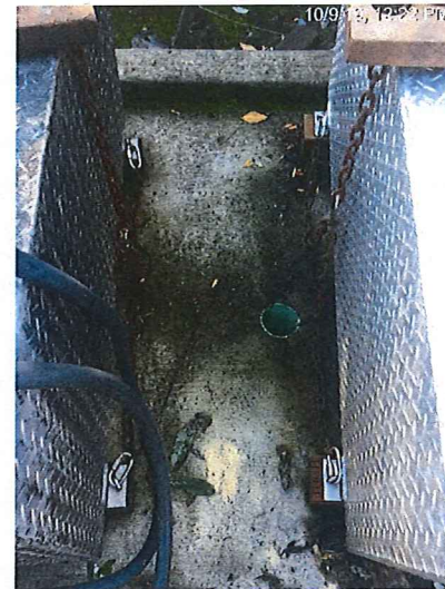
02 DESCRIPTION: DRAIN FROM CENTER OF CONCRETE PAD BETWEEN FUELING TANKS, LARGE SEDIMENT BUILDUP ON GROUND
