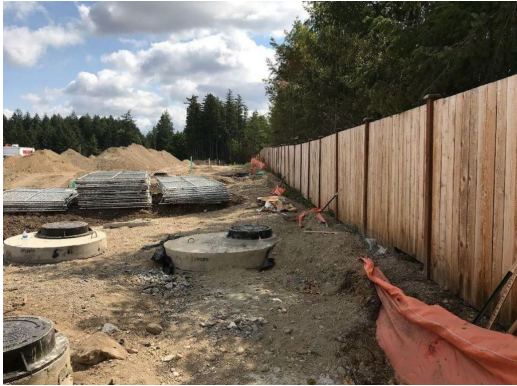
Ecology Photo 4: The section of silt fence must be repaired
