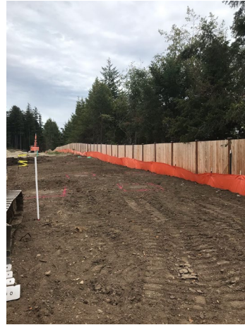
Lennar Photo 1: Section of silt fence repaired.
