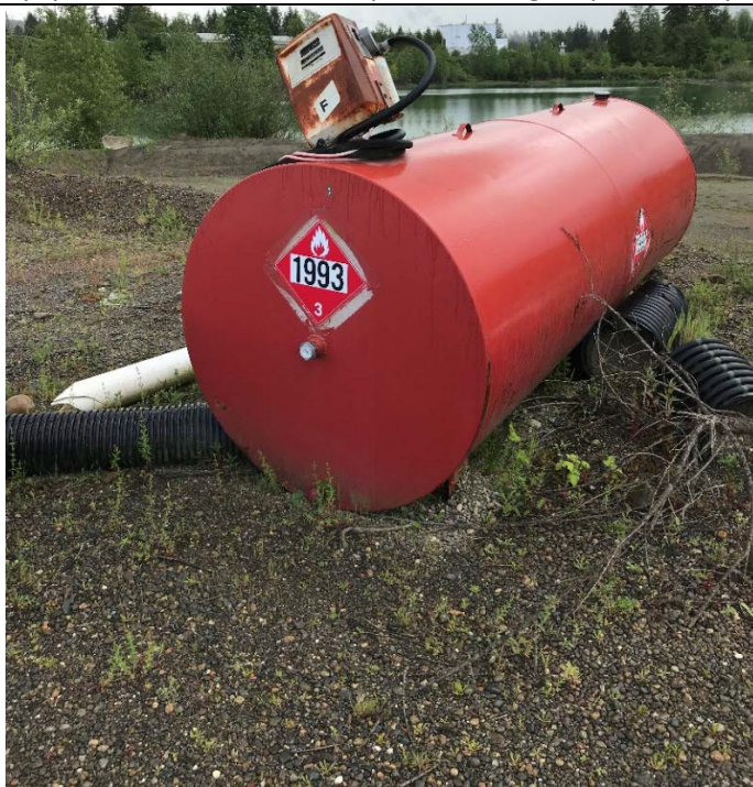
Photograph 6: Fuel tank with \frac{1}{4} full reading, not double-walled or in secondary containment.
