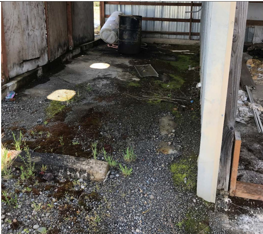
Photograph 3: Leaking drum labeled as chain oil, with secondary containment missing berm segment.
