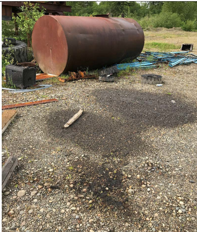
Photograph 1: Fluid spills on bare ground and tank not double-walled or in secondary containment
