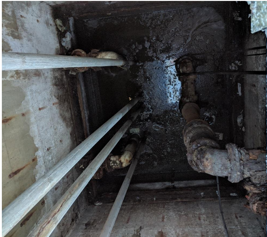
Photo No. 1: Piping corrosion in pump chamber (see Figure 2-4 for photo location).
