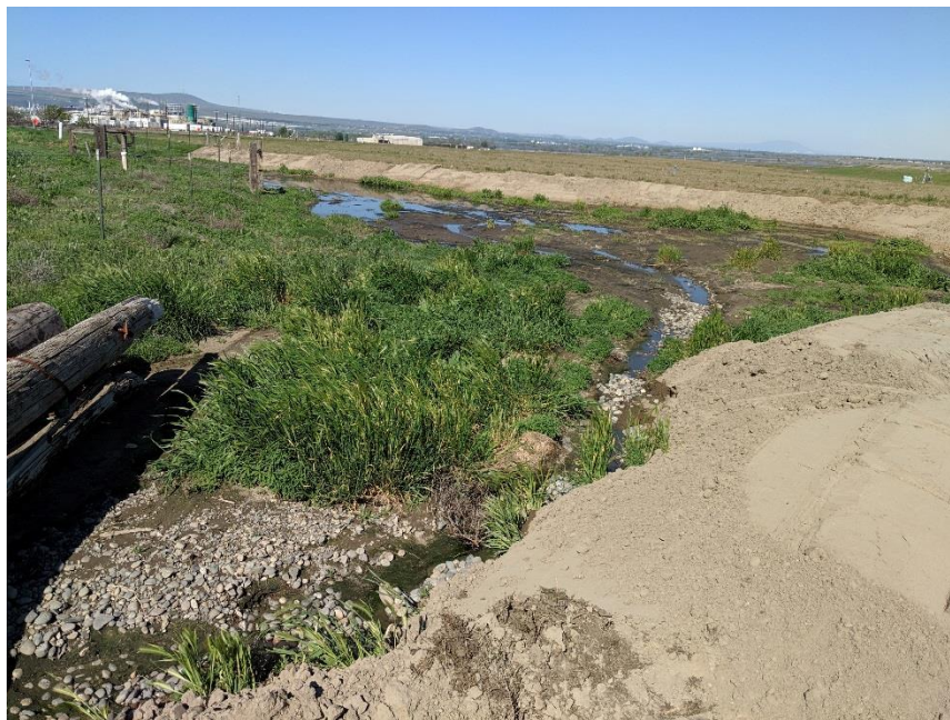
Photo No. 2: Partially treated sewage on the ground and plant growth on the north side of Absorption Bed No. 1 (see Figure 2-5 for photo location).
