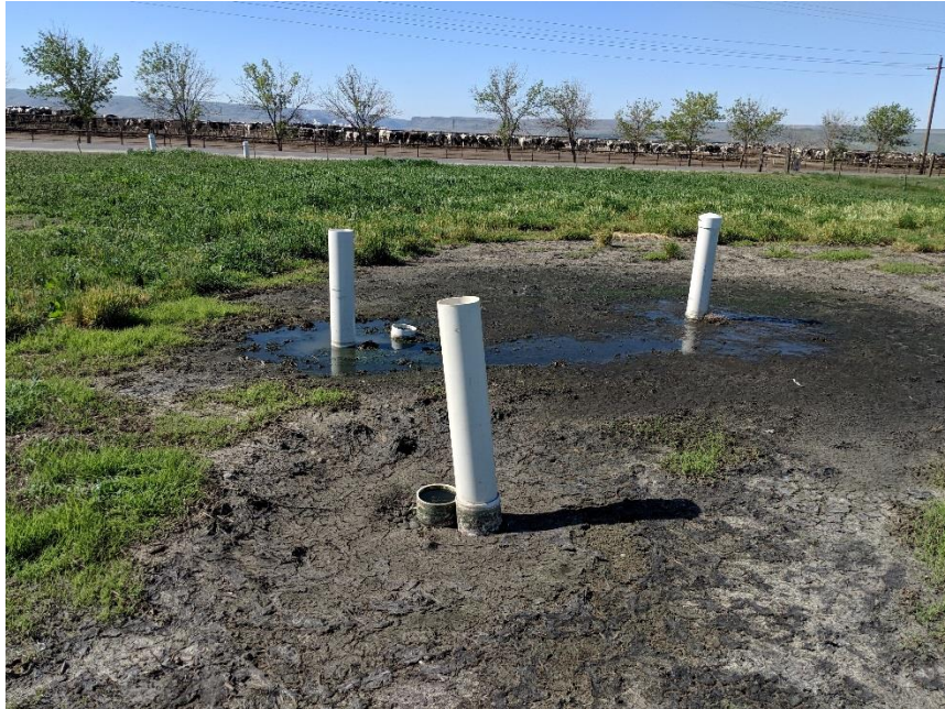
Photo No. 3: Partially treated sewage on the ground and plant growth at the center of Absorption Bed No. 1 (see Figure 2-5 for photo location).
