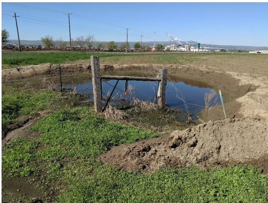
Photo No. 4: Partially treated sewage on the ground on the west side of Absorption Bed No. 2 (see Figure 2-5 for photo location).
