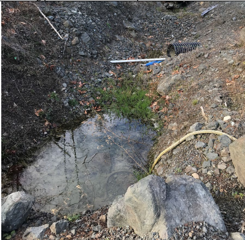
Photograph 2: Upper infiltration pond with pump hose and cross drain for routing to the G001 conveyance ditch
