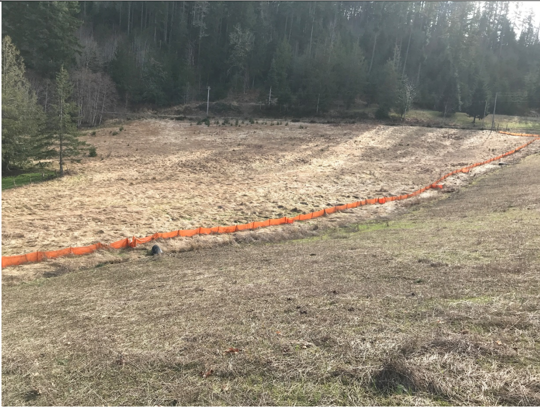
Photograph 3: Overflow pipe outlet and silt fence Best Management Practice (BMP)
