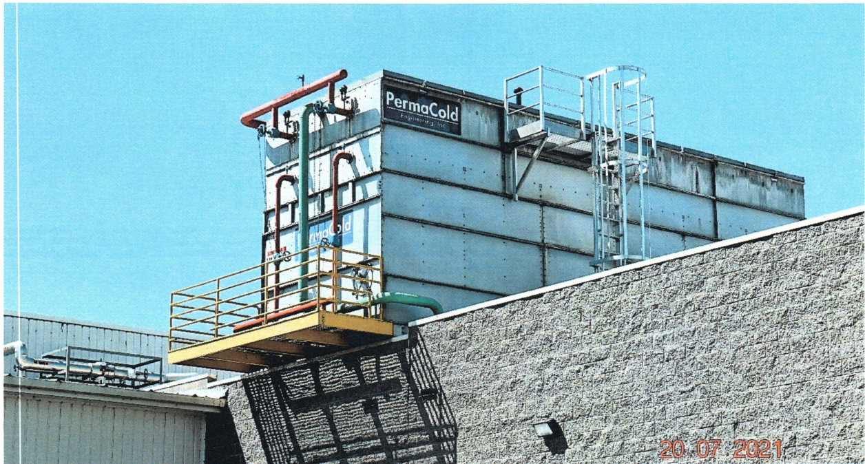
Figure 9-condenser units with regulation sump below
