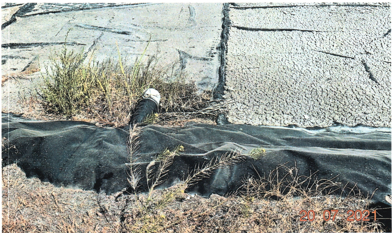
Figure 6- typical discharge pipe from evaporative cooler ice defrost discharge
