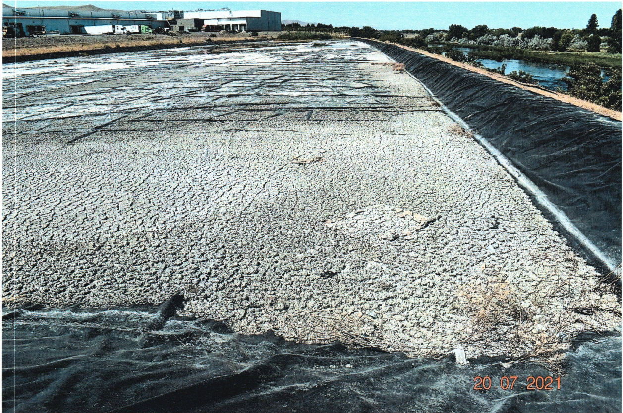
Figure 5-NE corner sediment, bird feces and debris accumulation
