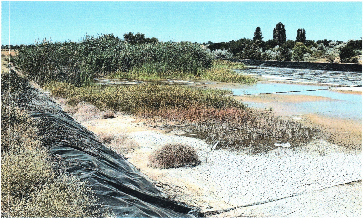
Figure 7-accumulated sediment and vegetation SW corner of pond
