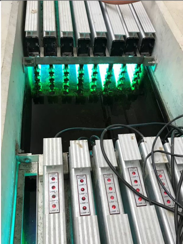
Date: 8/19/21 Taken by: G. Lipnickey Description: UV disinfection channel
