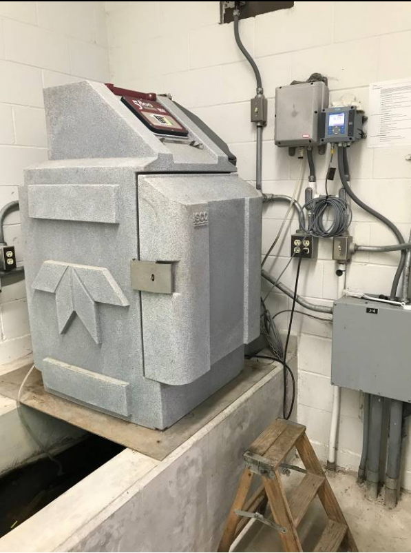
Date: 8/19/21 Taken by: G. Lipnickey Description: Effluent composite sampler
