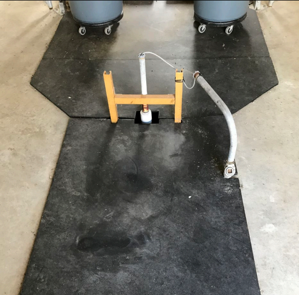
Date: 8/19/21 Taken by: G. Lipnickey Description: Floor-mounted influent flow meter
