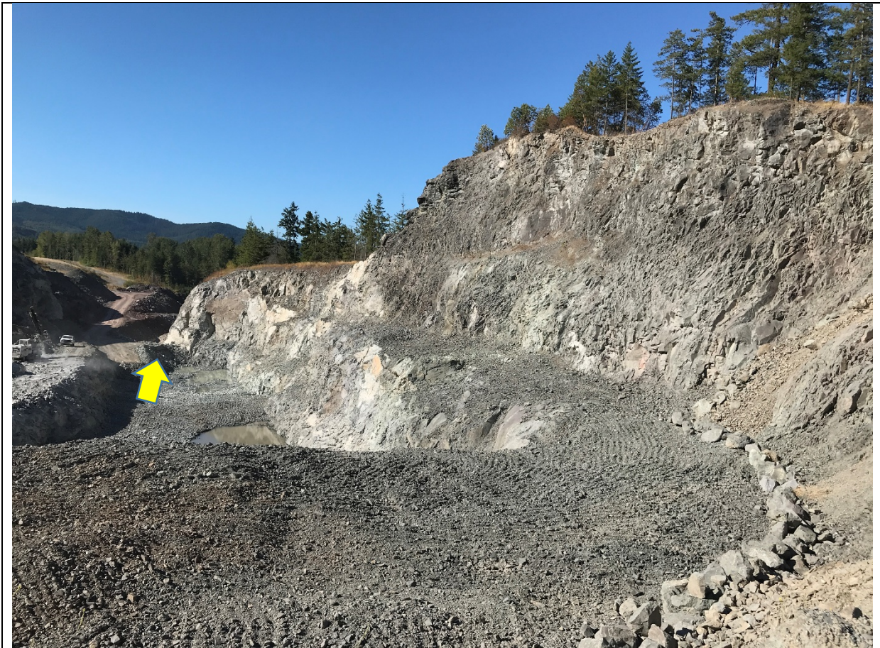
Photograph 4: Overblasting in quarry floor directs stormwater to the infiltration pond.
