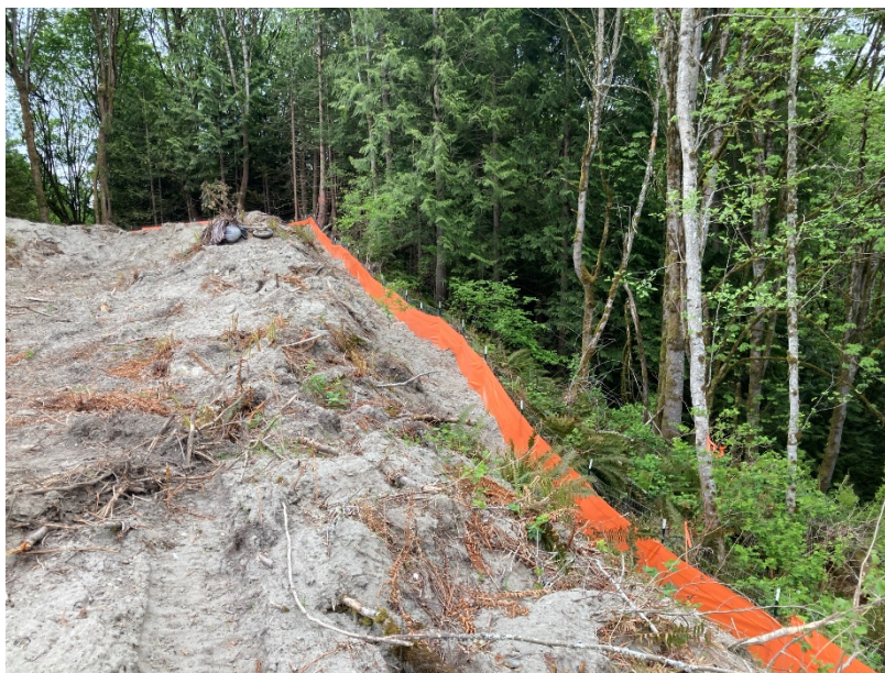
Figure 10 Description: The CESCL must evaluate sediment accumulation along silt fence. Maintain the silt fence as required in BMP C233. Remove sediment deposits when the deposit reaches approximately one-third the height of the silt fence, or install a second silt fence. Stabilize exposed and unworked soils as required in Condition S9.D.5.d.
