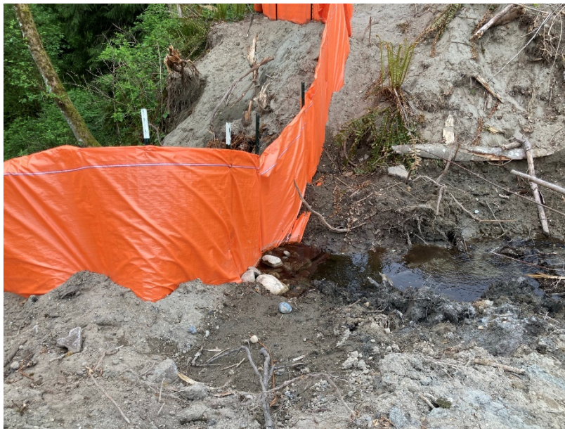
Figure 6 Description: Stream 1 discharge from limits of disturbance down a steep ravine. Stream 1 is tributary to Stream 2. The permittee must sample stormwater discharges occurring here until they achieve permanent stabilization, as required in S4.C.3.a.
