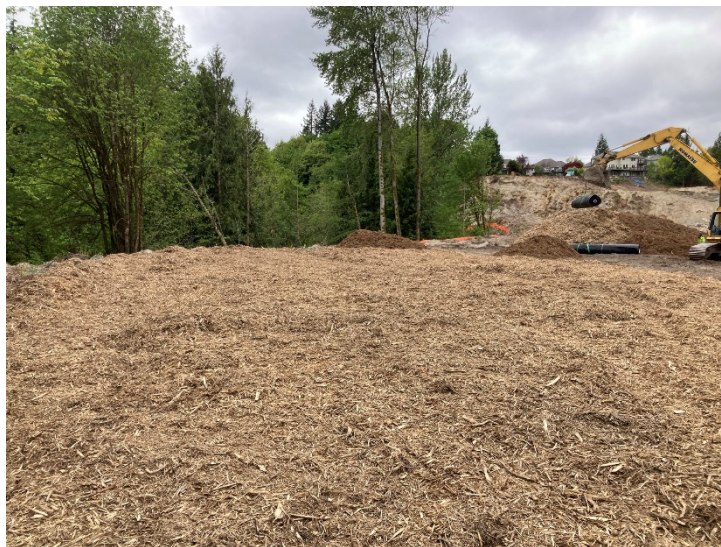
Figure 9 Description: Wood mulch stabilizing exposed soils.
