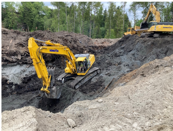
Figure 11 Description: On-going removal of landfill materials from the “wedge”.
