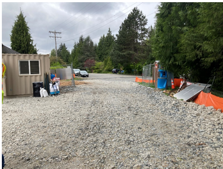
Figure 1 Description: Recycled concrete aggregate used to stabilize on-site road. This material may cause elevated levels of pH in stormwater runoff.
