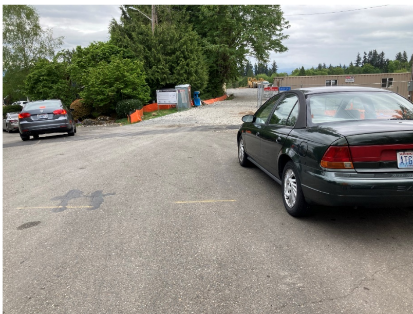
Figure 14 Description: Slight track out on to 108 th Street. Maintain the construction entrance as required in BMP C105. Clean 108 th Street thoroughly at the end of each day or more frequently as necessary, as required in Condition S9.D.2.d.
