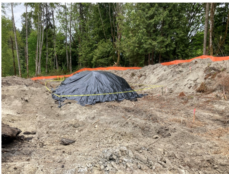
Figure 12 Description: Stockpile covered with plastic. Initial screened suggested asbestos contamination.
