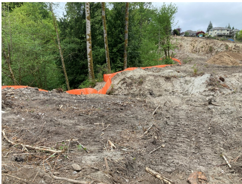
Figure 8 Description: Exposed and unworked soils without stabilization BMPs for more than 7 days as required in S9.D.5.d.
