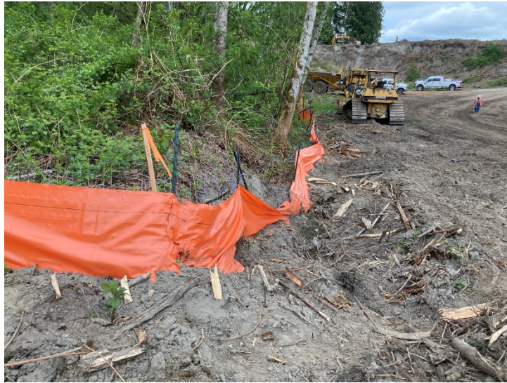
Figure 5 Description: Overall silt fence remained in good condition; however, this section needs repair.
