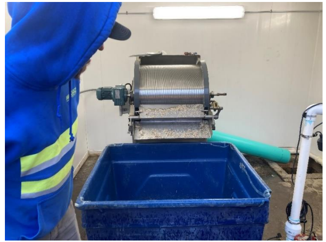
Photo 8 Description: New rotating self-cleaning screen.
