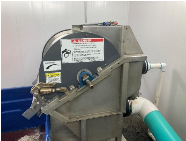
Photo 9 Description: Side view of new rotating screen.
