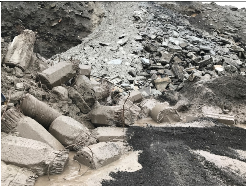
Photograph 6: RAP covering concrete sludge and discharge to groundwater.
