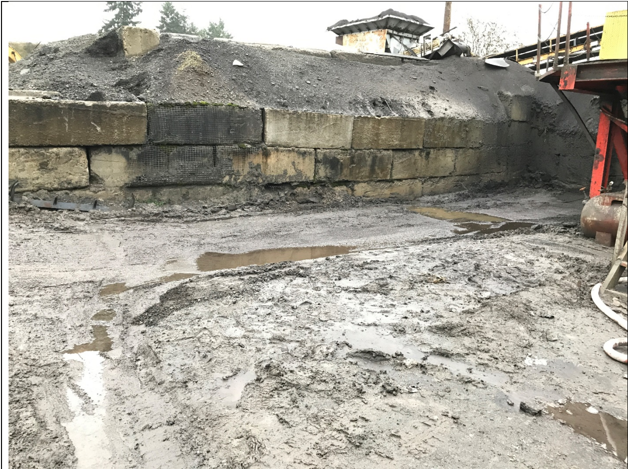
Photograph 4: The cement slab below the sludge has been exposed after by-product/sludge removal. Runoff from the remaining sludge is measured at a pH of 10.80 S.U. on the lined conveyance.
