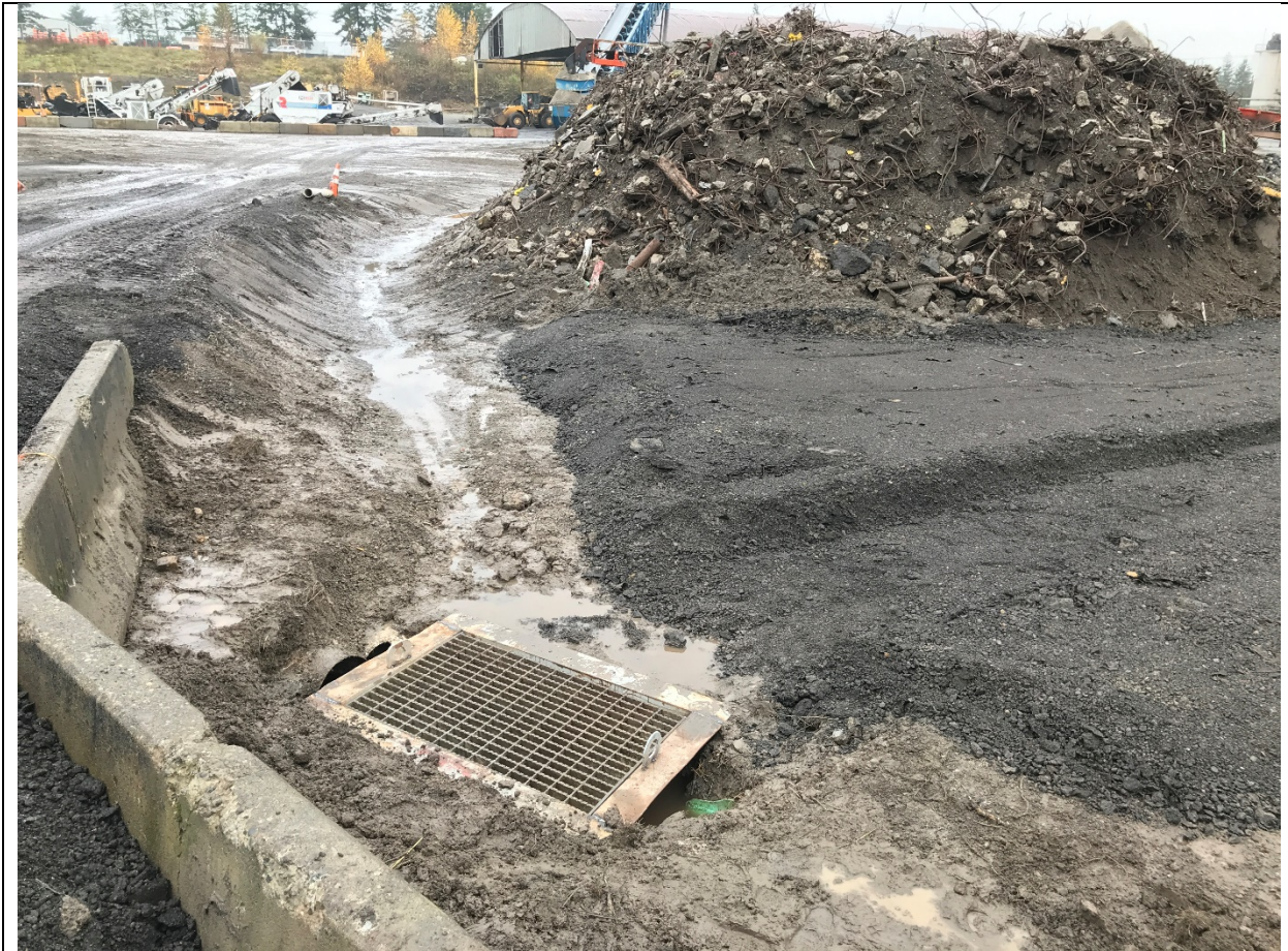
Photograph 2: The catch basin previously buried by concrete recycling by-product and sludge has been uncovered. Additional impervious surface and lined channel conveyance needed.
