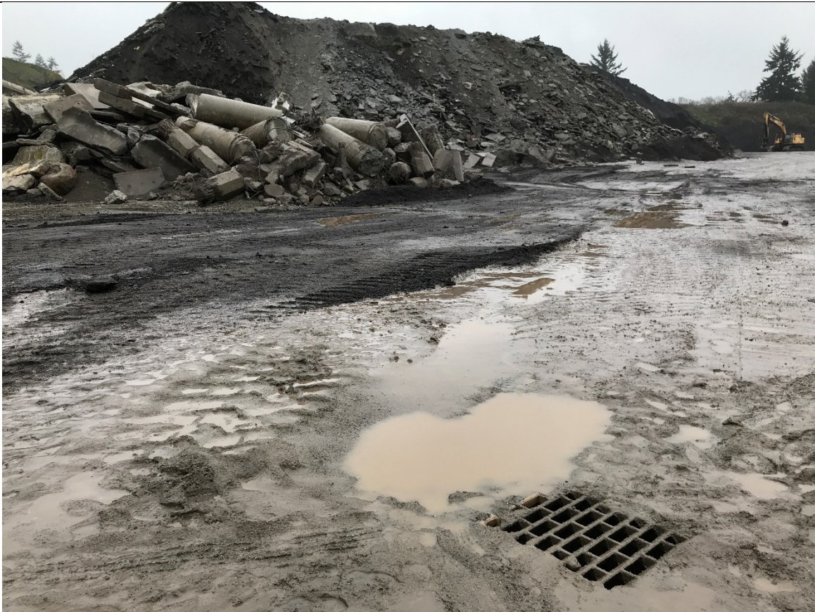
Photograph 8: Runoff from the concrete stockpile depression area is not contained by an impervious surface or lined channel conveyance to the catch basin.
