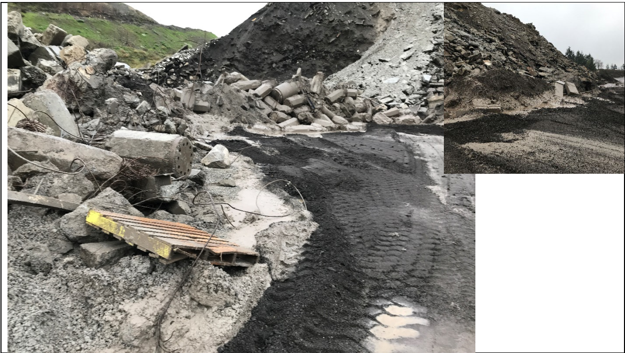
Photograph 5: The base of the concrete stockpile has been partially covered with recycled asphalt product (RAP). Concrete sludge and unhardened concrete are observed on the bare ground. The discharge to groundwater is measured at pH 11.83 S.U for monitoring point G003.
