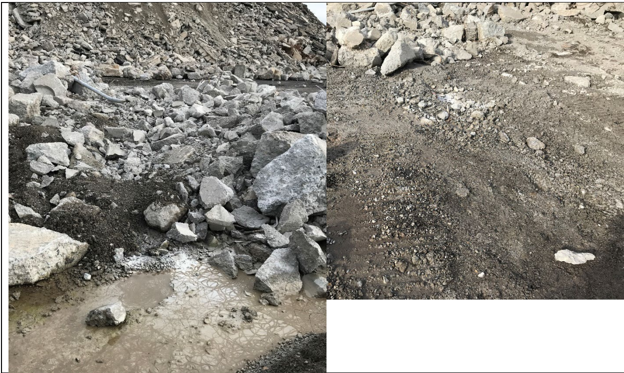
Photograph 4: Unhardened concrete, leachate, and discharges to groundwater remaining near the base of the concrete stockpile (monitoring point G003).
