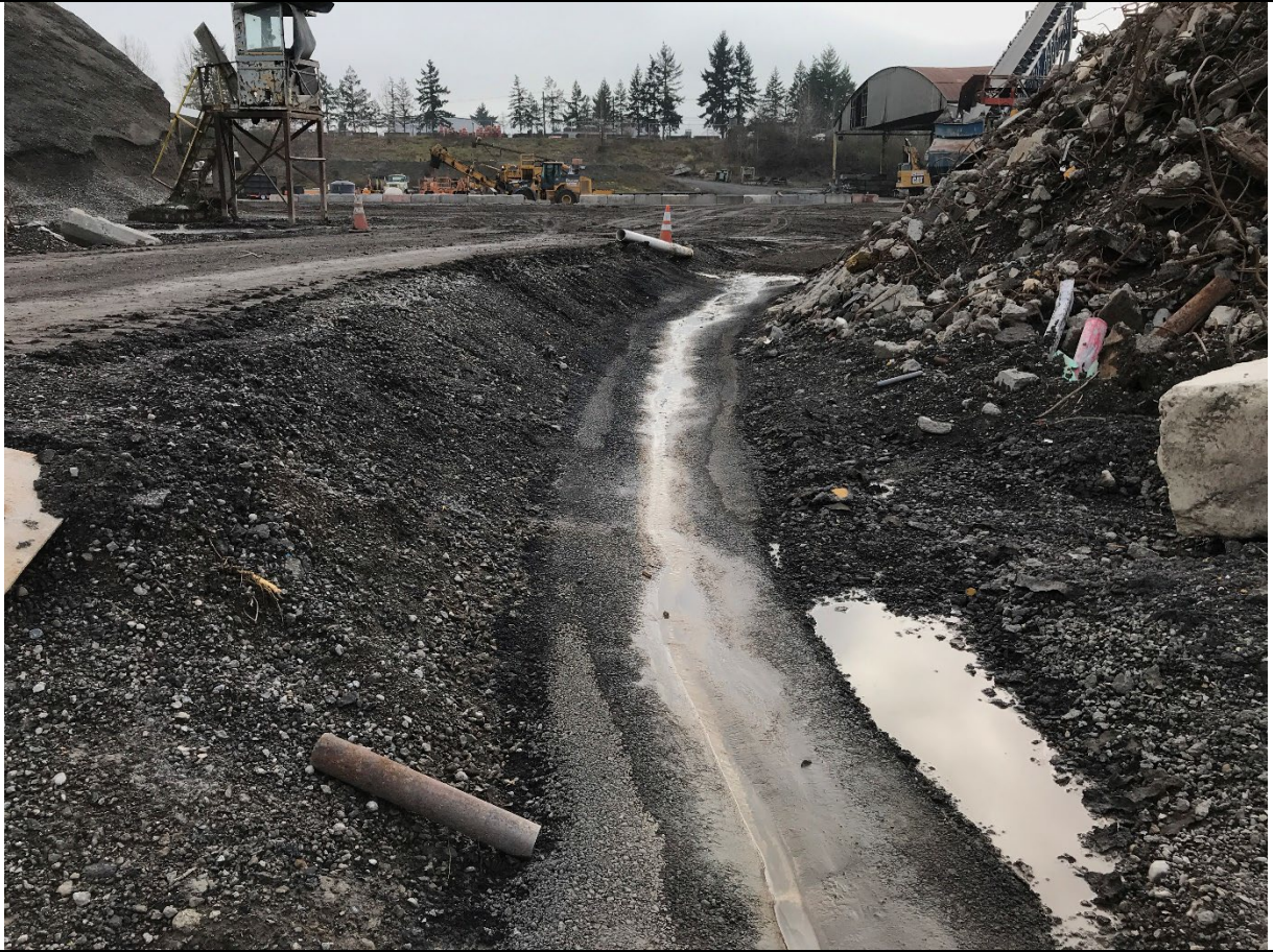
Photograph 1: Asphalt lined conveyance.
