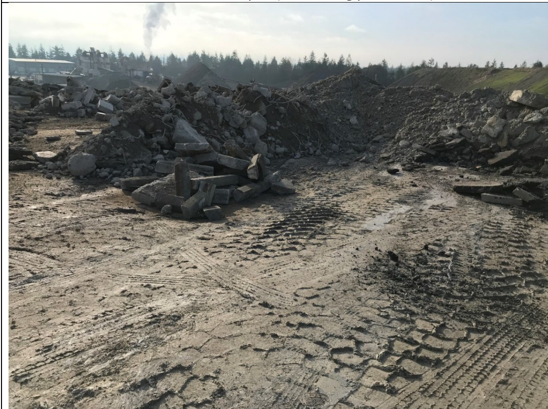
Photograph 5: Concrete sludge and unhardened concrete moved to the top of the stockpile.
