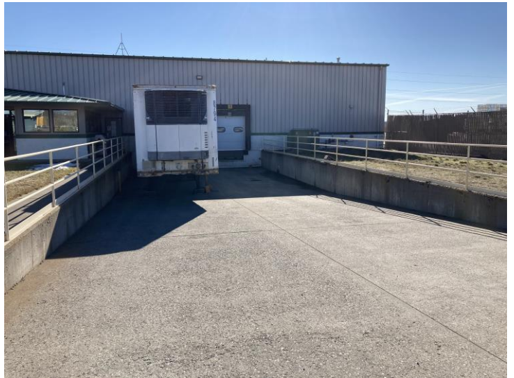
FIGURE 4: TRUCK LOADING BAY. ENTIRE INSIDE OF BUILDING IS PLUMBED TO DISCHARGE TO THIS LOADING BAY IN AN EMERGENCY SPILL SCENARIO.
