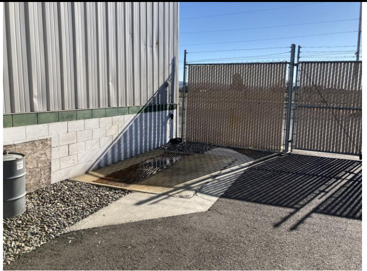
FIGURE 2: SMALL WASH BAY WITH DEAD-END SUMP FOR WASHING CONTAINERS.
