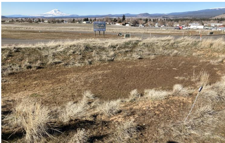
FIGURE 5: STORMWATER INFILTRATION POND. DISCHARGE PIPE REMAINS CAPPED, FOR EMERGENCY USE ONLY.
