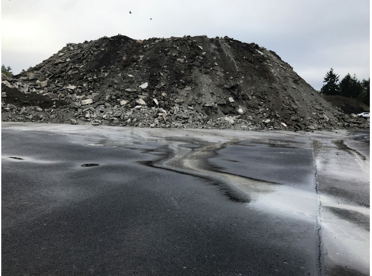
Photograph 1: Asphalt paving conveys concrete pile runoff to the catch basin.
