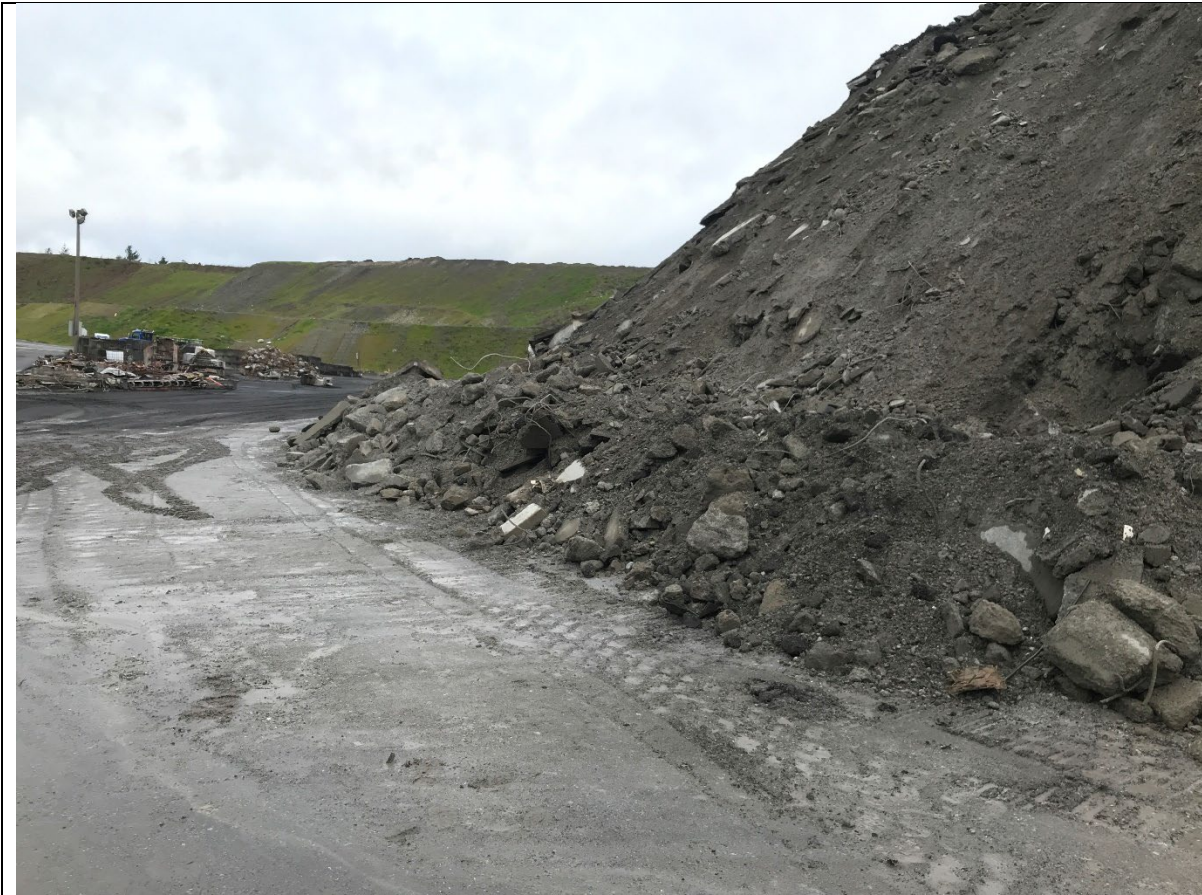
Photogrpah 2: Unpaved areas that do not currently contain ponding water. As the concrete pile is recycled, asphalt should extend under the pile to convey all runoff to the lined system and prevent future discharge violations.
