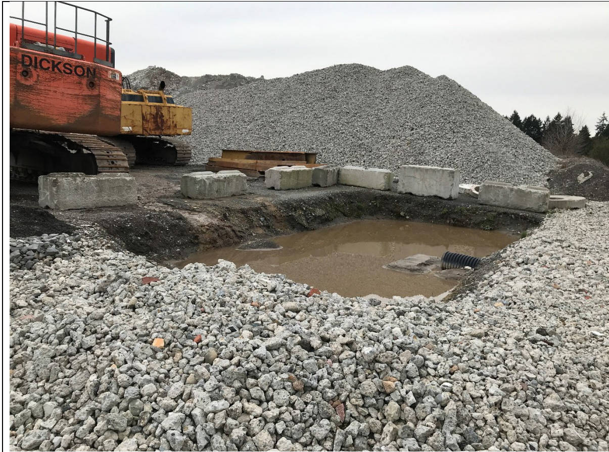
Photograph 4: Impoundment in bare ground where runoff from the concrete crushing and stockpile area is collected before being piped to the main infiltration pond. I measured a pH of 11.57 S.U. in this pond.
