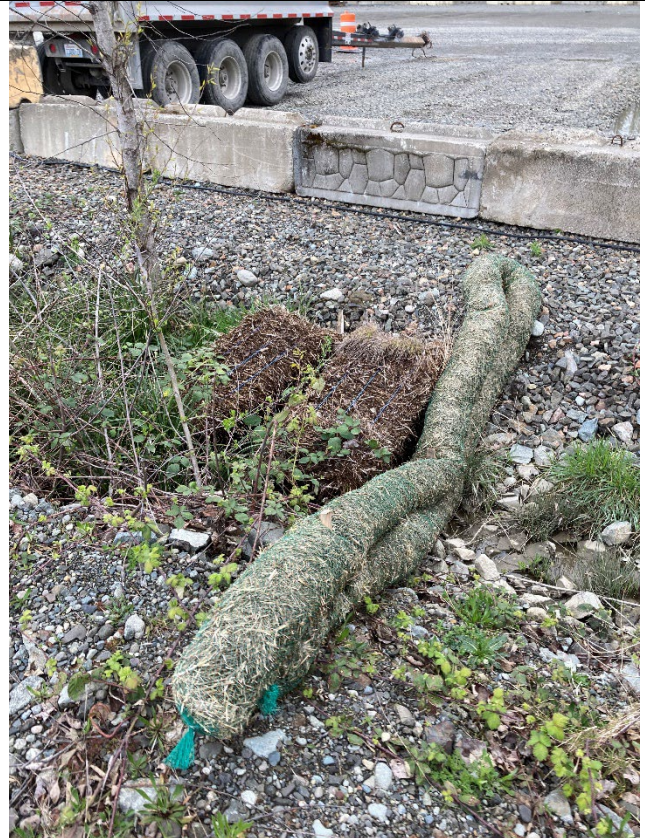
Photo 44 Description: Photo of straw wattles and bales.
