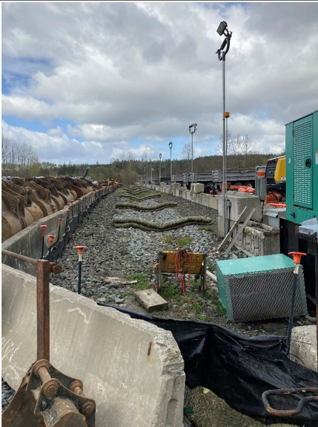
Photo 43 Description: Facing west, photo of rock-lined ditch with silt fences and wattles.
