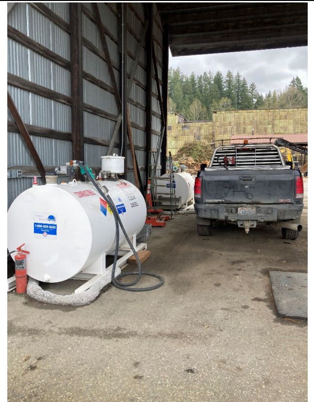
Photo 16 Description: Photo of fueling station with no drip pans.
