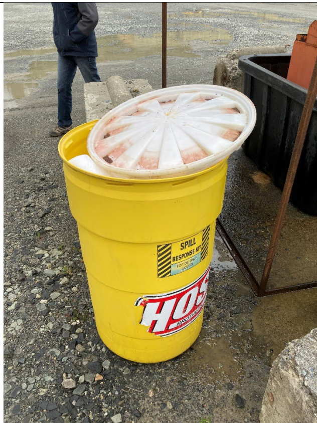
Photo 30 Description: Photo of spill kit next to fuel tank.
