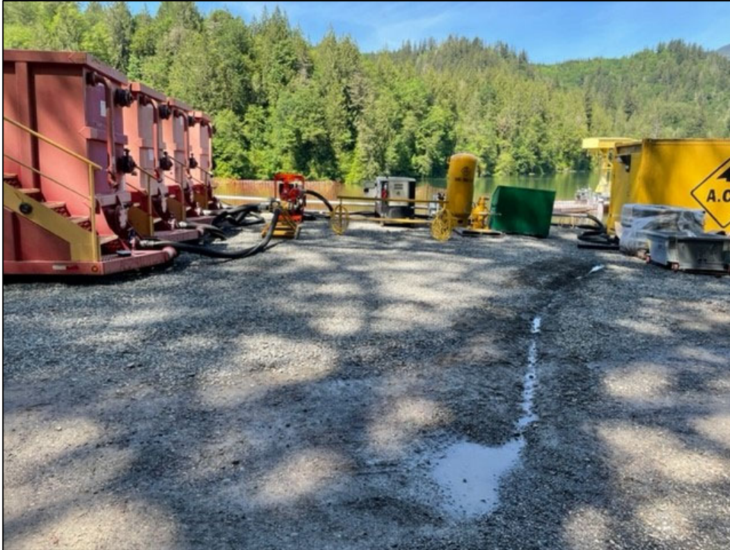
Figure 5. BR-1 on June 6, 2022; construction road leading to boat ramp; hand-dug ditch installed in the construction access road to divert stormwater back onto the construction site.
