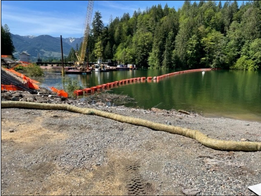
Figure 4. BR-1 on June 6, 2022; boat ramp with straw wattles installed across the width of the top of the ramp.
