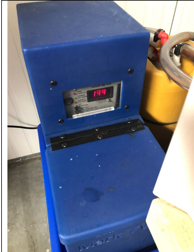
Photo 5: Silver recovery unit for photo processing wastewater discharge point SP007.
