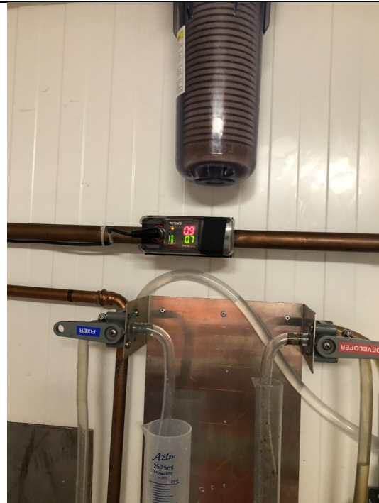
Photo 4: Flow meter for photo testing discharge point.
