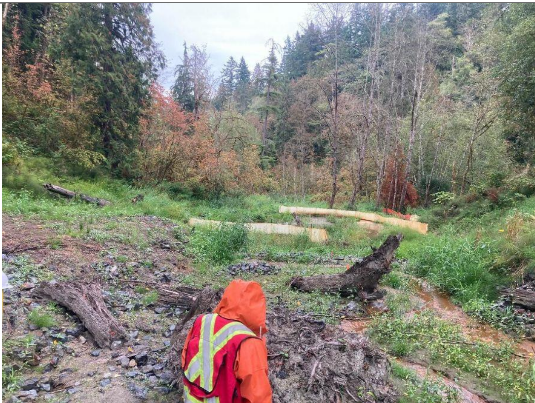
Photo 2 Description: Discussed silt fence j hook extension and straw wattle checks refreshed in this area of the slide.
