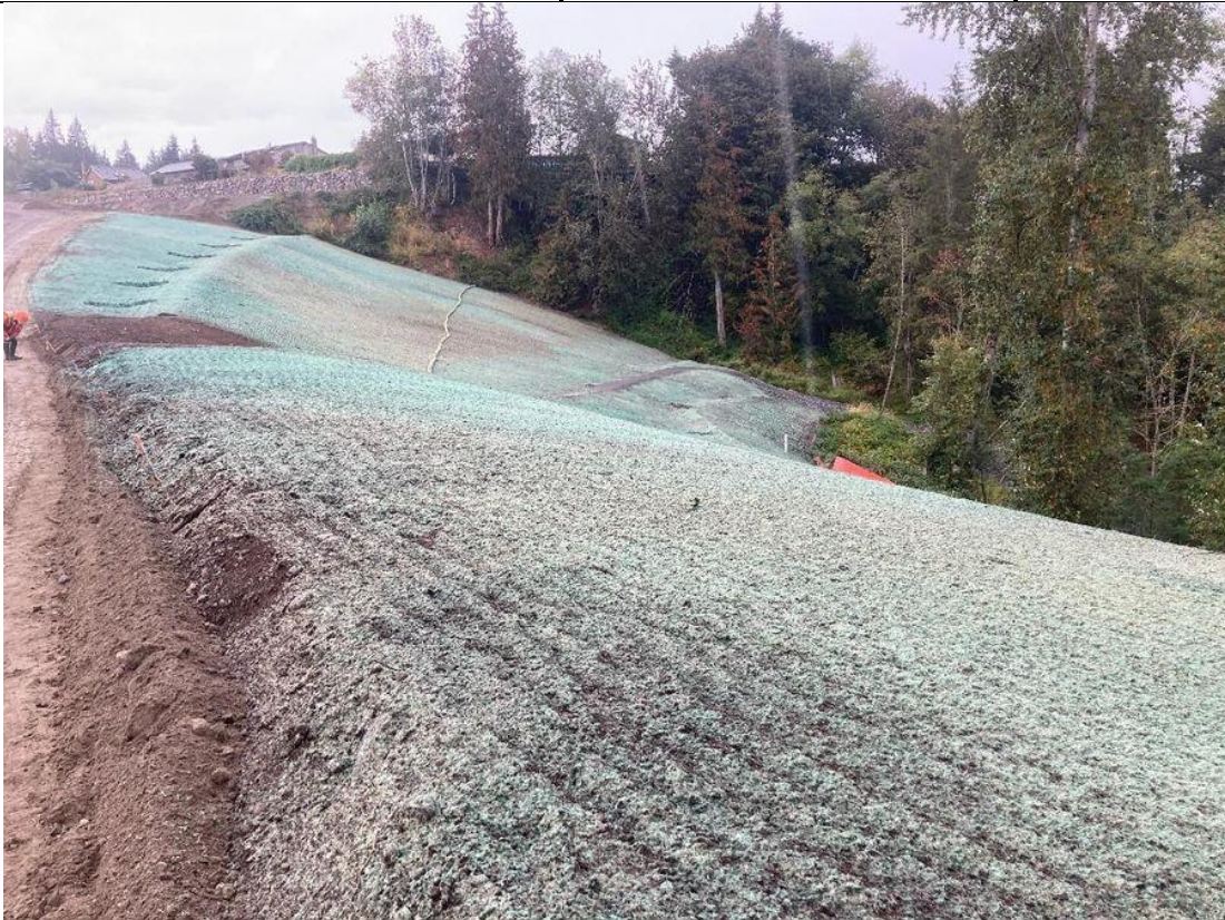
Photo 7 Description: Slope above slide was hydroseeded.
