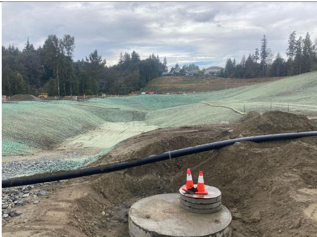
Photo 8 Description: Pond and slopes above hydroseeded.
