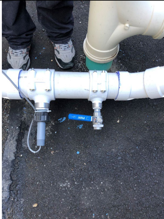
Photo 8: Effluent pH meter and sample port of discharge line.
