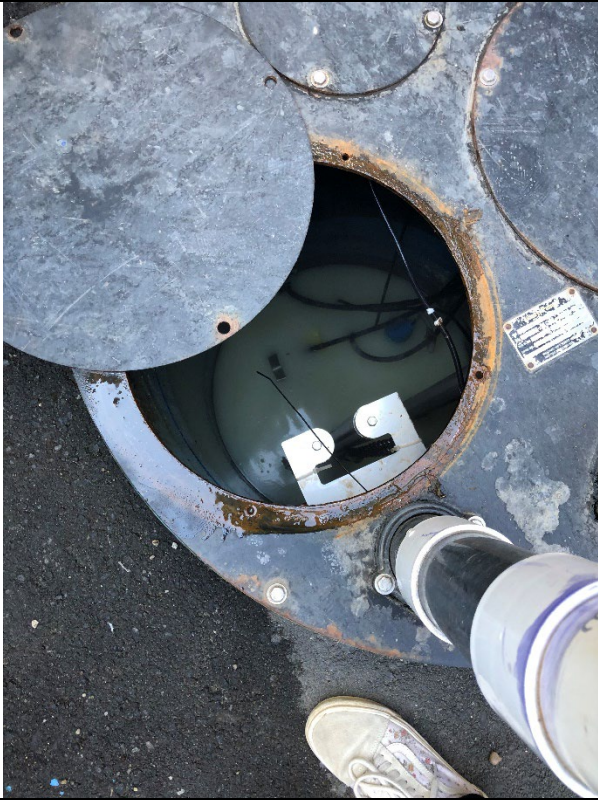
Photo 5: Wastewater sump after grease interceptors. Wastewater is pumped from this sump to the pH neutralization tank.
