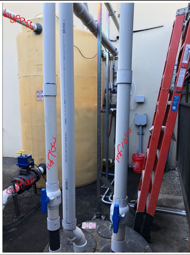
Photo 10: Piping orientation of pH neutralization tank (inflow, outfall, and bypass noted).
