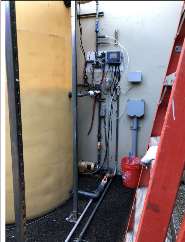
Photo 9: Larger perspective photo of recirculation line, controller, and pH neutralization tank.
