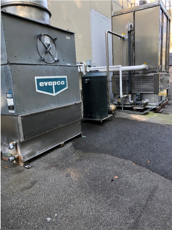
Photo 13: Cooling tower system. The smaller green tank is an overflow tank for the system that collects city water.
