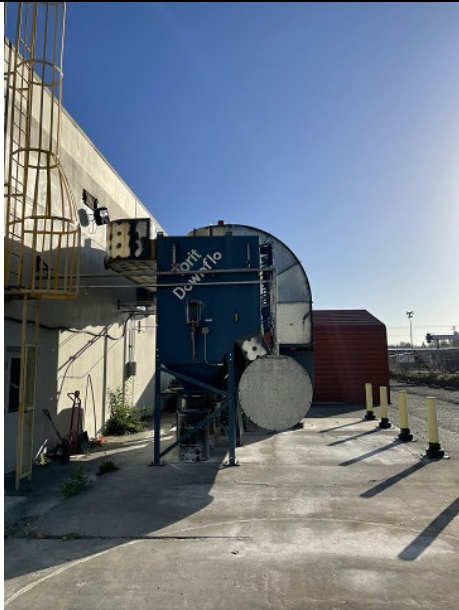
3. Cyclone dust collection system at west end of south side of 1010 building
