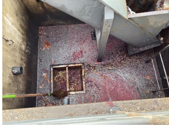
Drain under auger arm with screen
