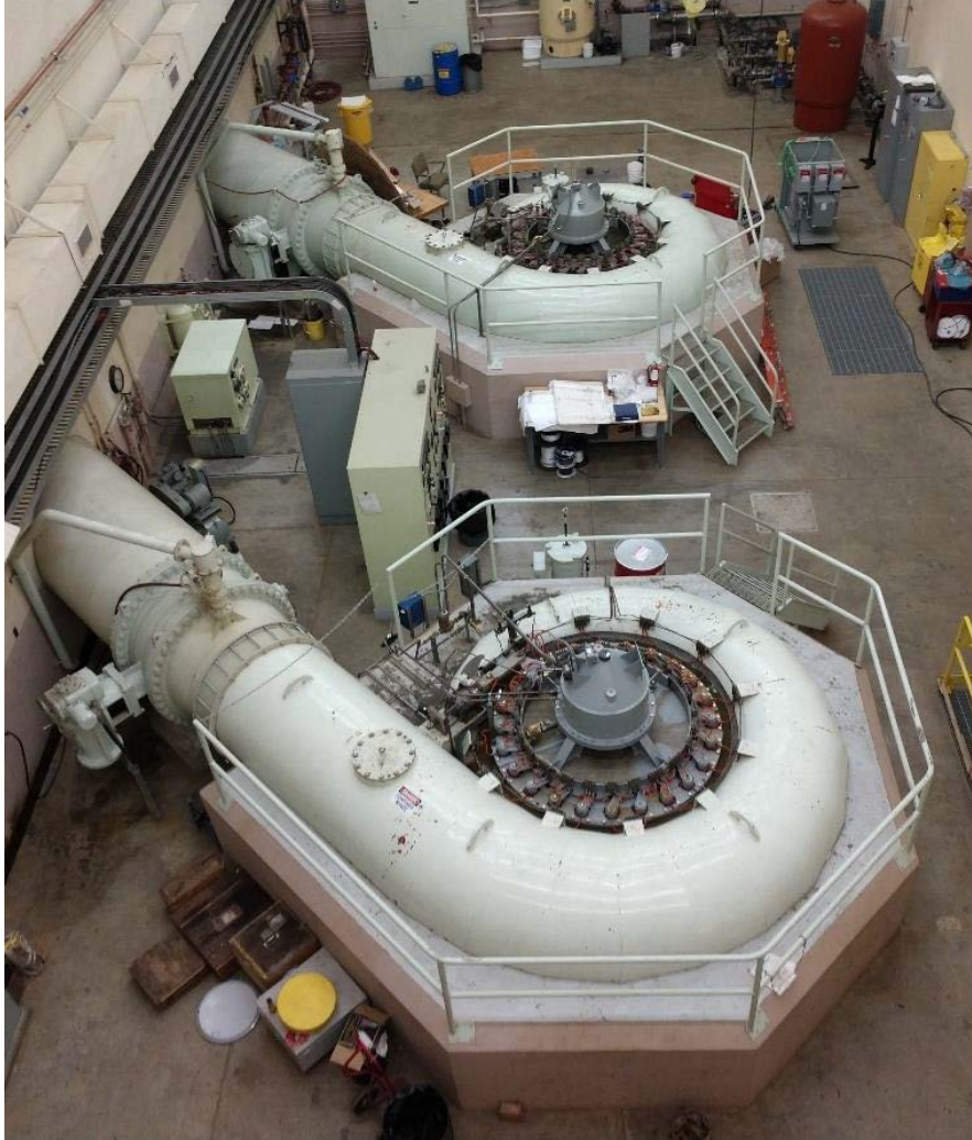
Figure 3 The Wanapum Dam fish attraction water pumps are being used for in-house testing of the two EAL greases that met the compatibility tests qualifications. Due to their small size, and the yearly maintenance, Grant PUD decided that testing on the fish attraction water pumps was the best course of action to identify any wear issues or compatibility problems.
