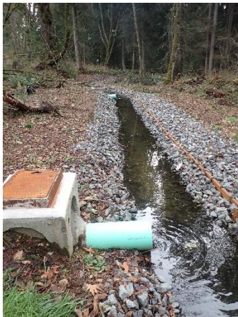
PHOTO 7 FLOW CONTROL AND DISPERSION SYSTEM
