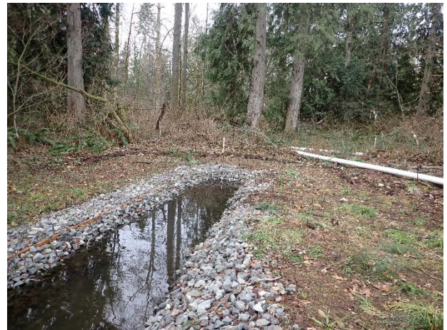
PHOTO 8 FLOW CONTROL AND DISPERSION SYSTEM
