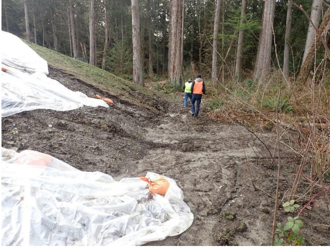
PHOTO 5 EVIDENCE OF EROSION AT THE BOTTOM OF THE SLOPE.
