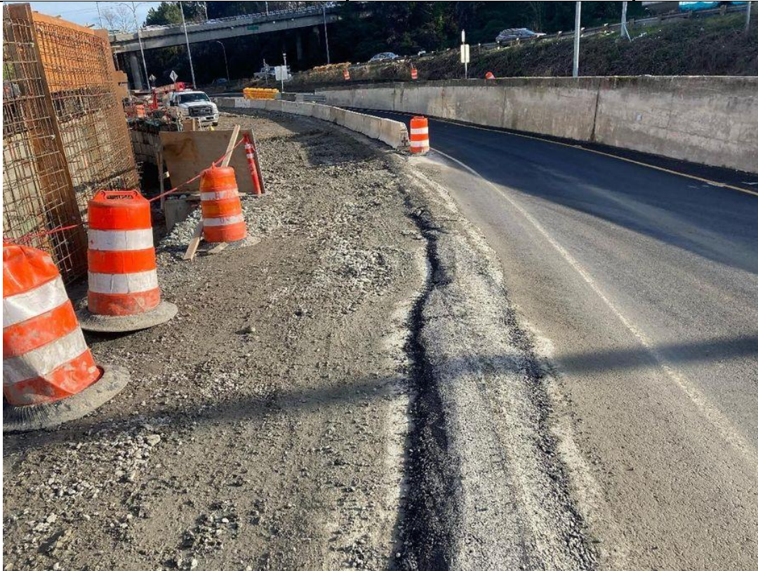
Photo 1 Description: Minor track out observed. Maintain exit as needed.
