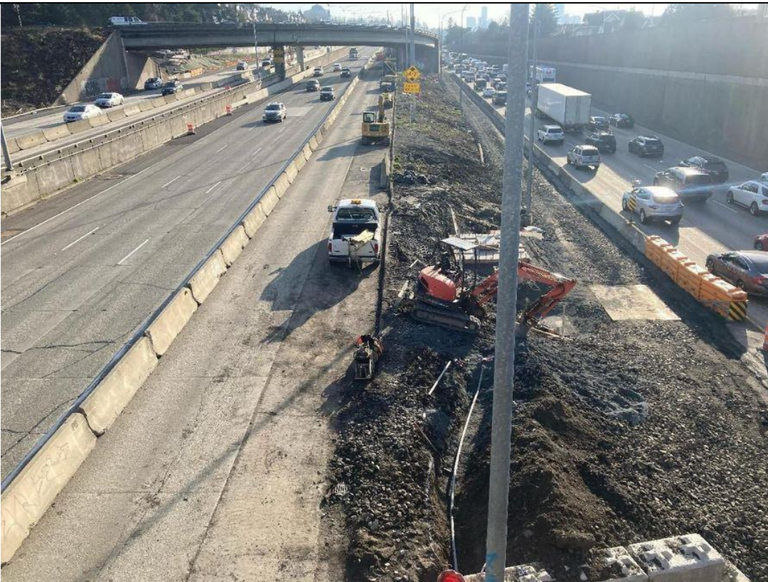
Photo 2 Description: Access road had no BMPs to direct any sediment flows towards a sump.
