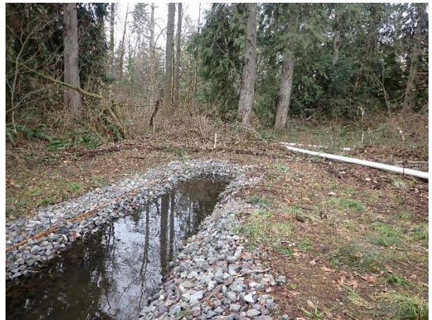
PHOTO 8 FLOW CONTROL AND DISPERSION SYSTEM
