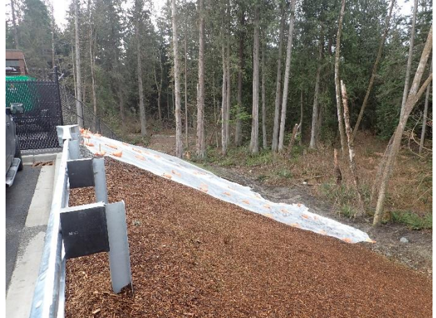
PHOTO 4 WEST SLOPE. THE IS EVIDENCE AT THE BOTTOM OF THE EROSION OF THE SLOPE. COSNTRCUTION COMPANY APPLIED BARK AND PLASTIC SHEETS FOR EROSION CONTROL.
