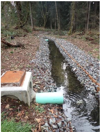
PHOTO 7 FLOW CONTROL AND DISPERSION SYSTEM
