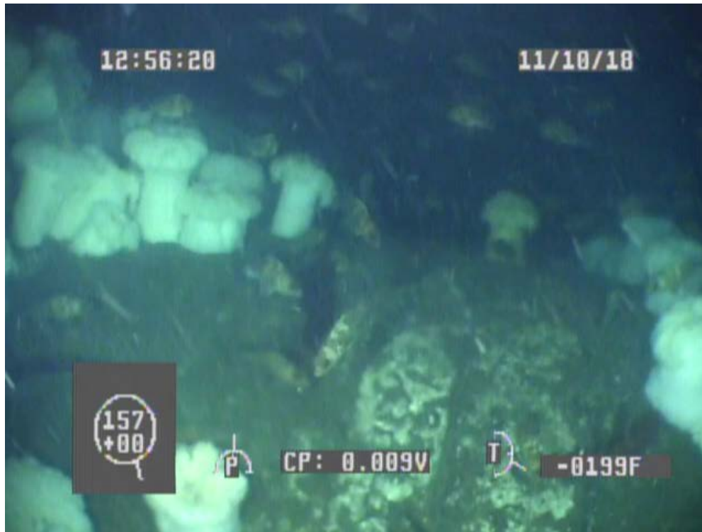
Figure 11: Leaking joint offshore of manhole number 8. This is looking at the crown and 11 o'clock position on the north side of the pipe. Effluent was observed leaking from the joint just below this image. Note the dark spot in the center of the screen just to the left of the joint is a piece of kelp, not a hole in the pipe.
