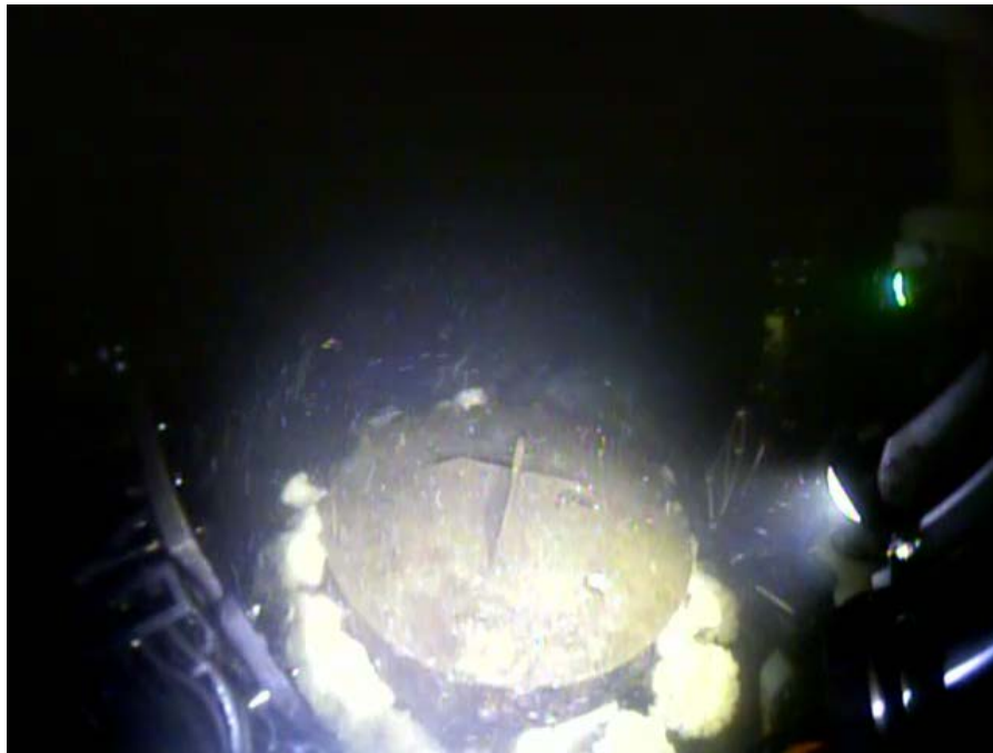
Figure 12: Manhole 9, intact. The position of manhole number 9 was determined by checking that diffuser ports were still present below the manhole and verifying the approximate depth to the as built drawing.
