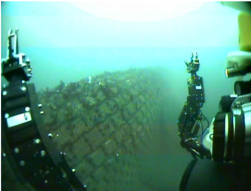
Figure 16 Mat over crown at outlet structure, typical
