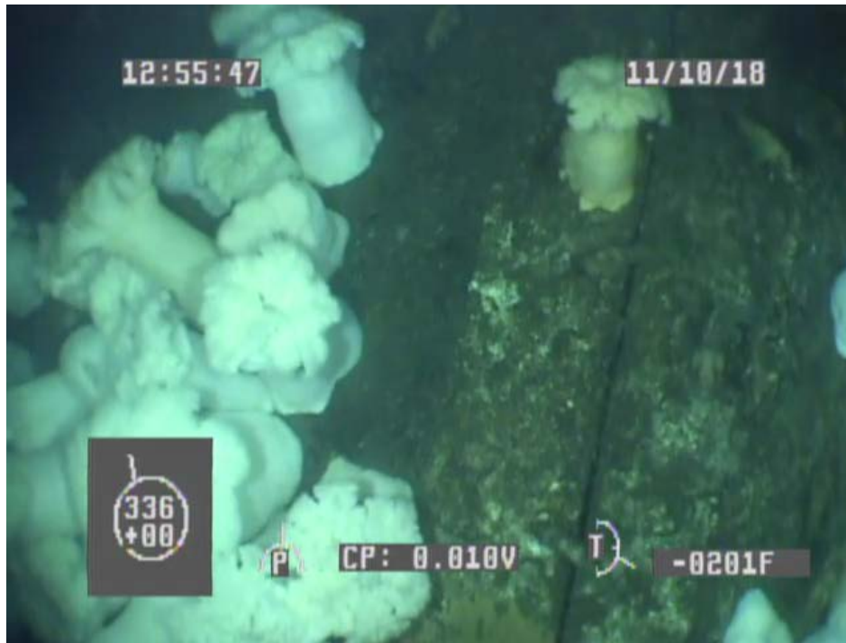
Figure 9: leaking joint offshore of manhole number 8 seen from the south side of the pipe. Note: no effluent was observed coming out of the seam from this location
