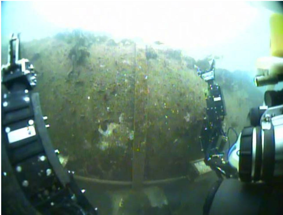
Figure 13 Wide angle view of loose band between brackets, no concrete mats
