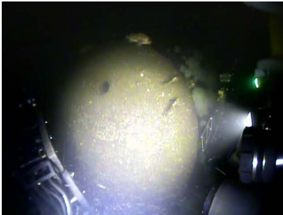
Figure 2: looking at the South half of the end gate. Note: a small amount of effluent exiting the diffuser port on the vertical centerline of the end gate
