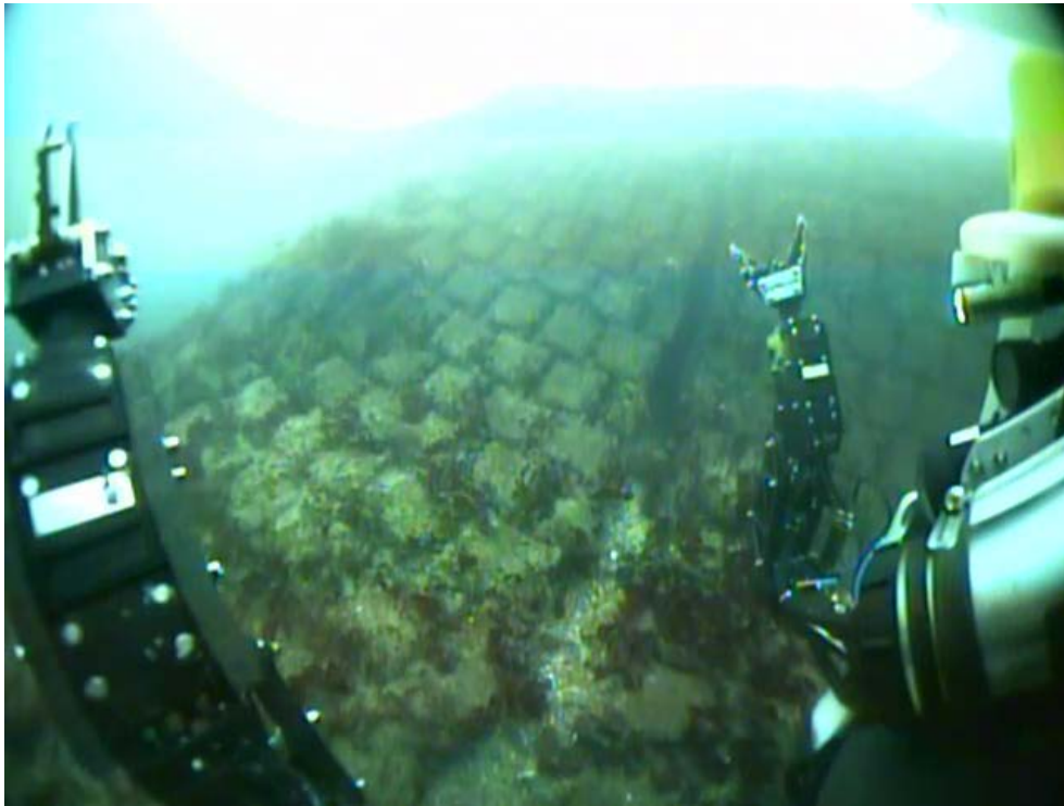
Figure 11 North side of pipe, typical condition, gap between mats
