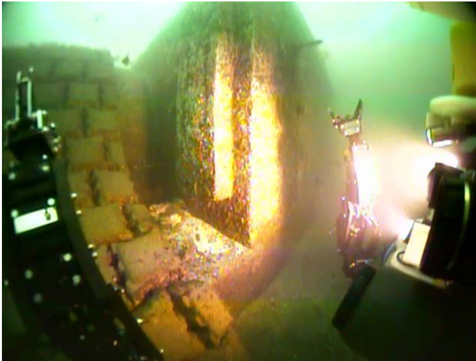
Figure 3 North side, concrete mat and outfall transition
