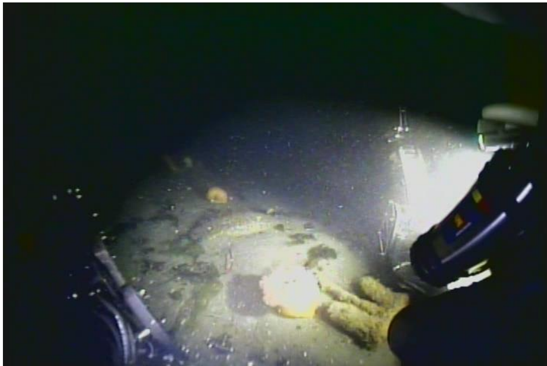
Figure 5 South Pipe, manipulator probe at joint. Note: Danforth anchor debris, lower right.
