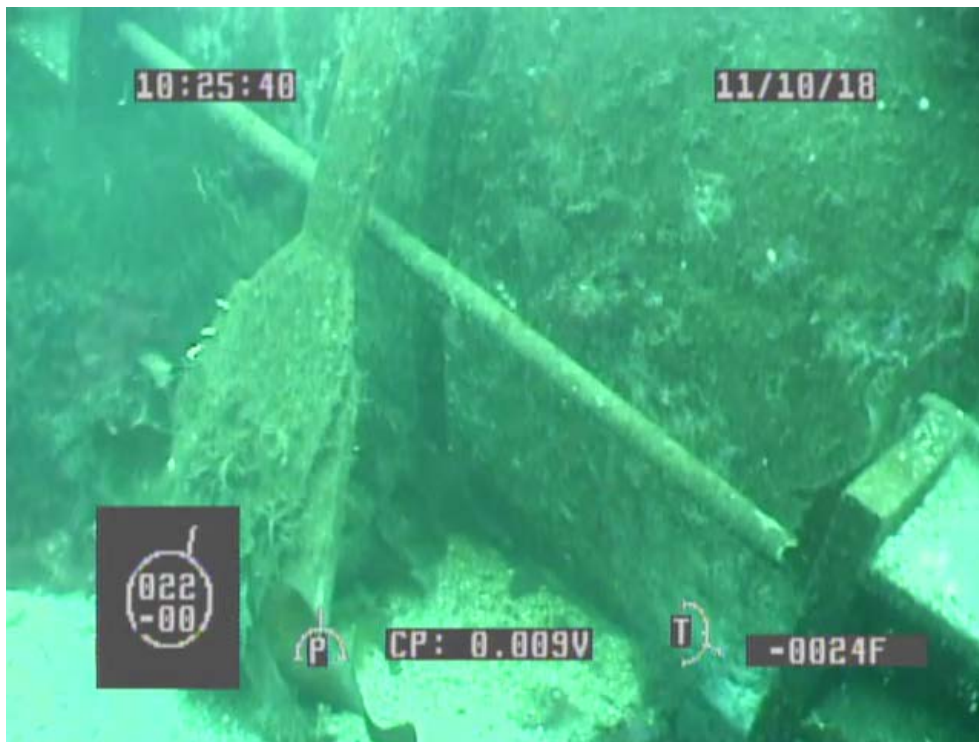
Figure 12 Loose tiebolt and band between brackets
