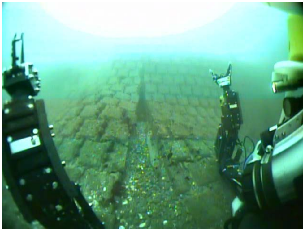
Figure 10 Gap between concrete mats
