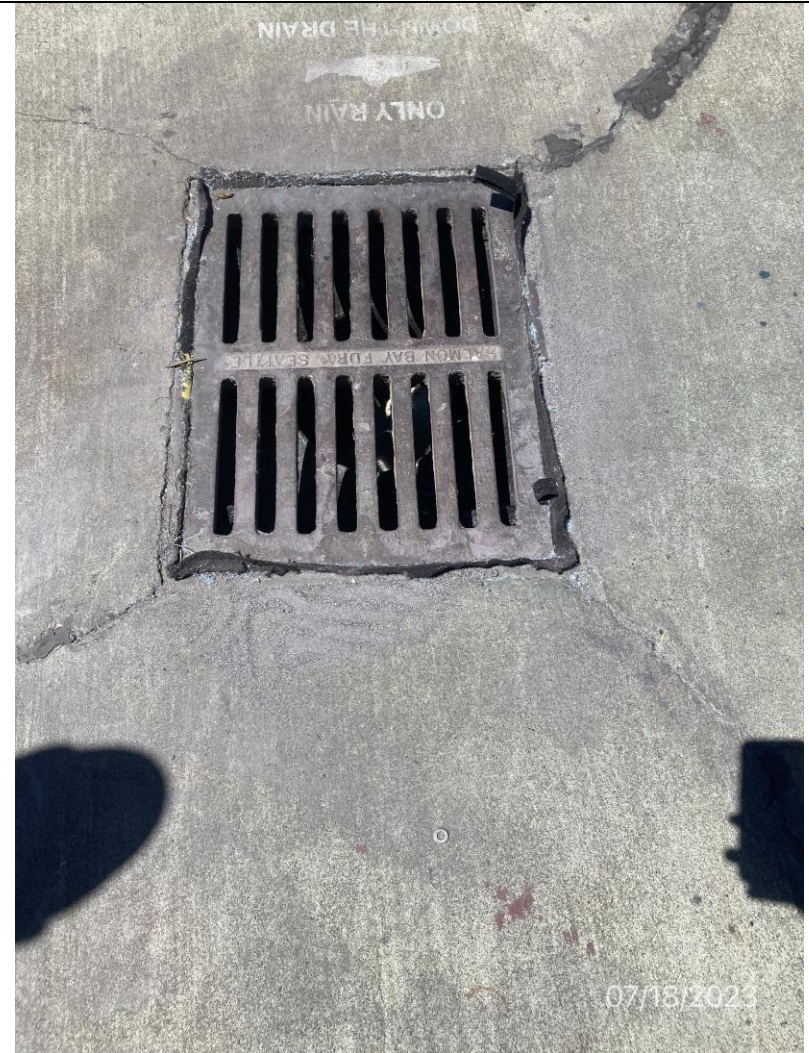
012 Description: Photo showing catch basin with insert. Large amounts of fine debris around this catch basin that is on the east side of the main building.
