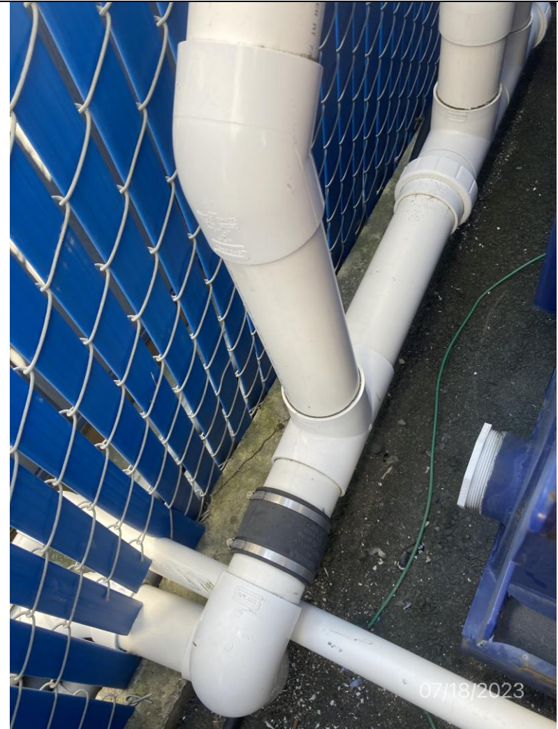
006 Description: Photo showing Stormwater-Rx piping after overflow connection where new sample port needs to be installed for permit compliant sampling.
