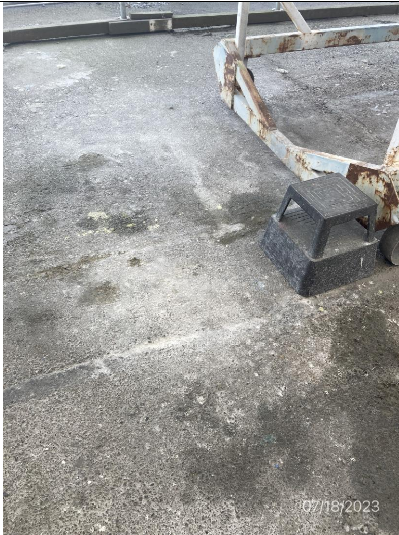
011 Description: Photo showing sanding dust on ground inside temporary tent structure due to not using tarping during vessel maintenance activities involving sanding of the exterior.
