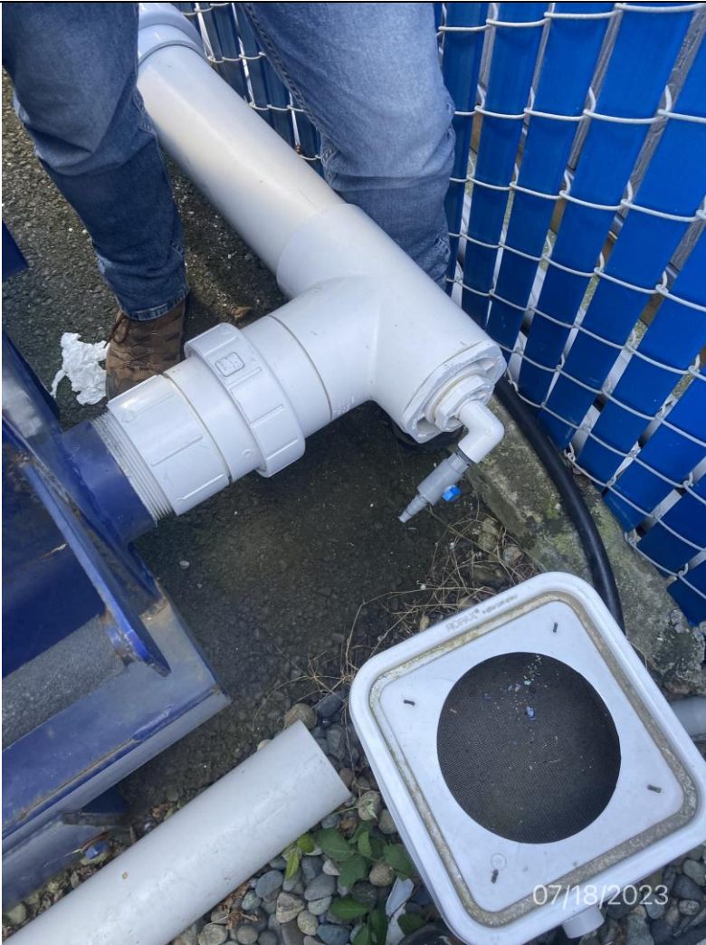
005 Description: Photo showing Stormwater-Rx current sample location which does not collect overflows.
