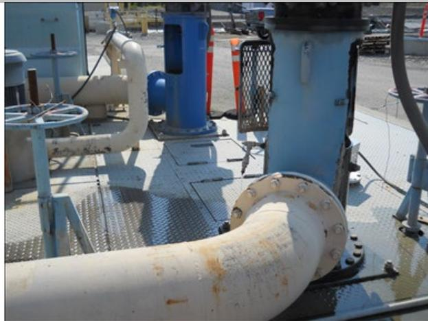
Photo 15: Castor oil pumps and feed system to walnut shell filtration system
