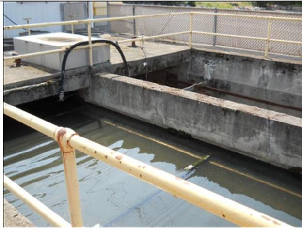
Photo 9: Trickling filter at the site's sanitary wastewater treatment system
