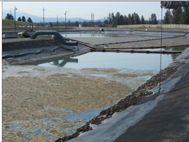
Photo 12: Wastewater settling lagoon. Algae/biological growth had formed on the pond surface. During the inspection, the facility was using a vector truck to collect the material and transfer it to their sludge drying lagoon.
