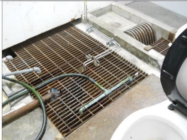
Photo 7: Ferric chloride and sodium hydroxide dosing setup used at the site's sanitary treatment plant. Ferric chloride is used to reduce phosphorus levels in the sanitary wastewater prior to discharge to the wastewater settling lagoon. Sodium hydroxide is used for pH control.
