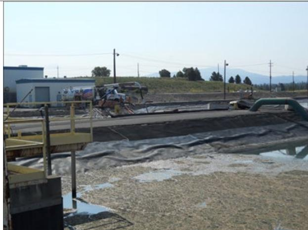
Photo 13: Hydrogen peroxide/UV treatment pilot system for PCB treatment located at the wastewater treatment area
