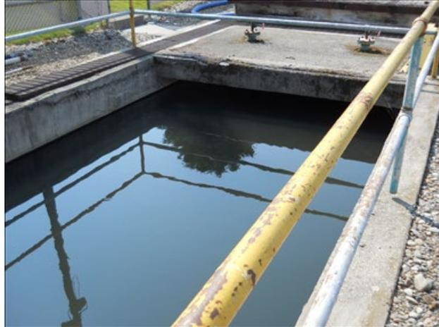
Photo 11: Wastewater settling lagoon
