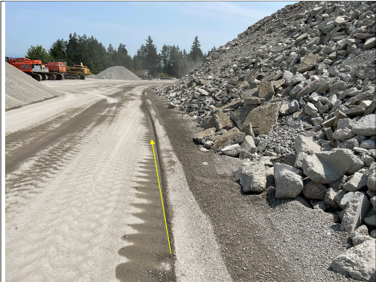
Photograph 2: Asphalt lined drainage path for concrete recycling related stormwater runoff (47.21681, -122.39281).
