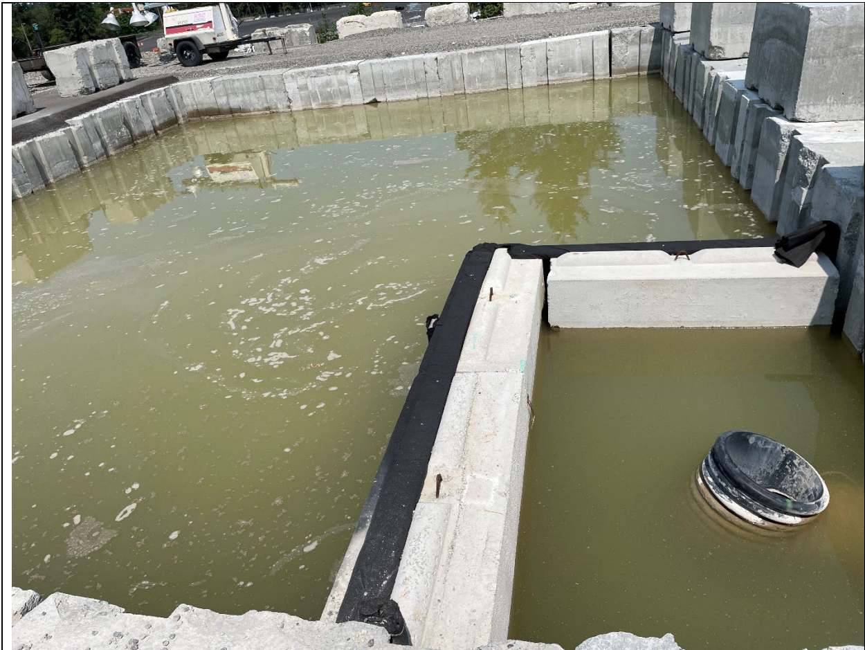
Photograph 4: Lined holding pond for concrete recycling related stormwater runoff (47.21697, -122.39118).
