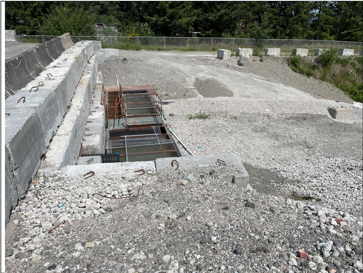
Photograph 5: pH treatment tank awaiting a CO2 treatment system installation (47.21694, -122.39107)
