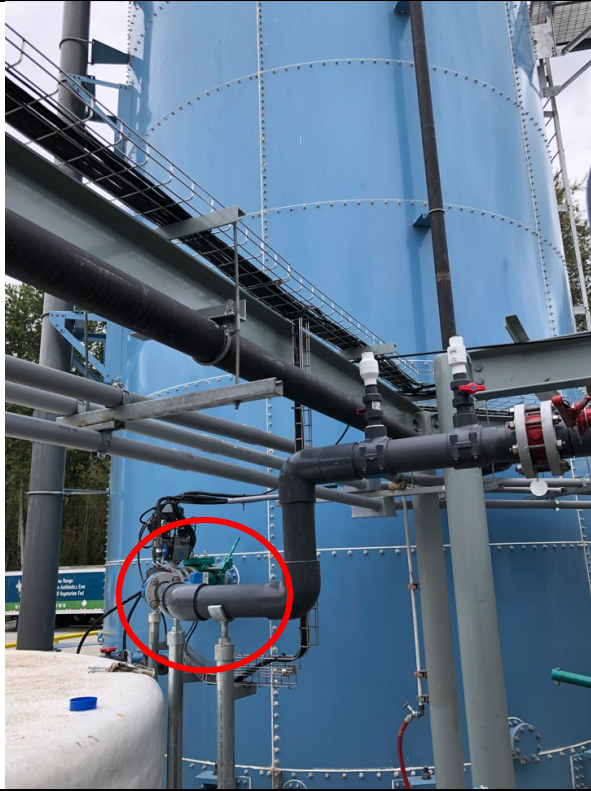
Photo 1: View of MBBR (blue tank), influent to MBBR noted by red circle
