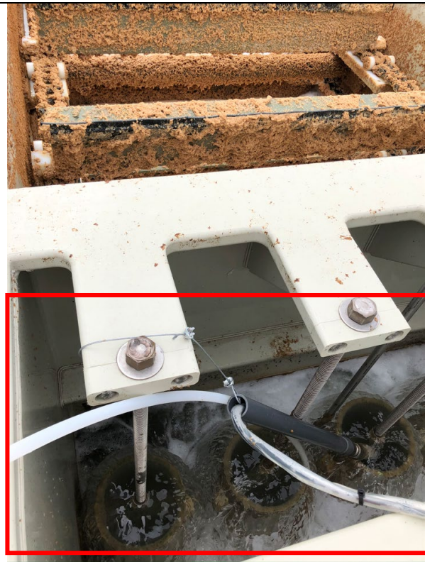
Photo 4: Secondary DAF effluent in foreground, noted by red box
