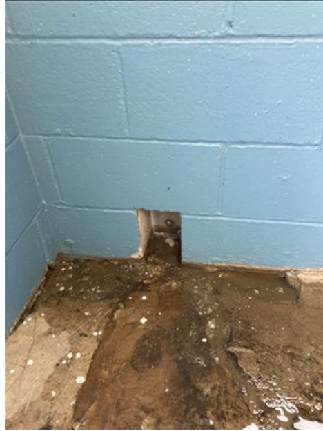
Photo 3. Building drain leading outside catchment
