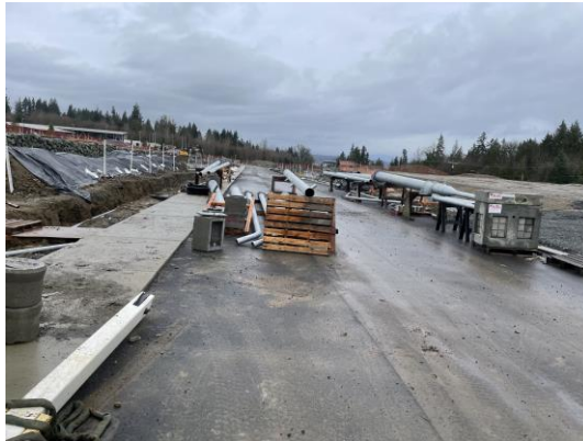
Figure: 8 Description: sidewalks in place. Soil on the road. BMPs covering the slopes on left side of the frame.
