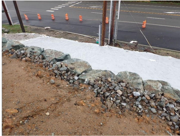
Figure 4 Description: outfall. Are of discharge from the vaults.
