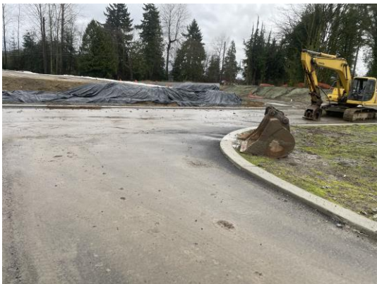
Figure: 15 Description: BMPs covering soils. Track out on road
