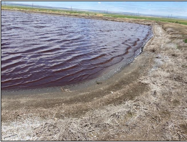
Photo 3. Wastewater lagoon with sludge covering liner.
