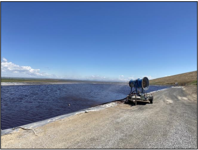
Photo 2. Wastewater lagoon with evaporator.
