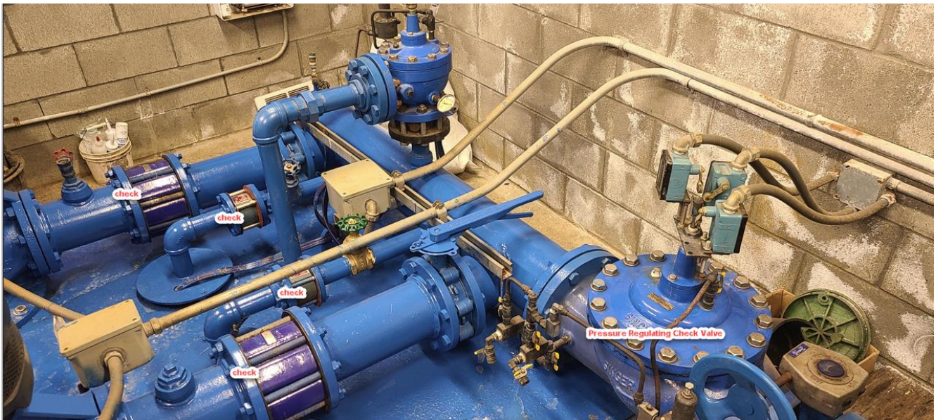
Pump house manifold
