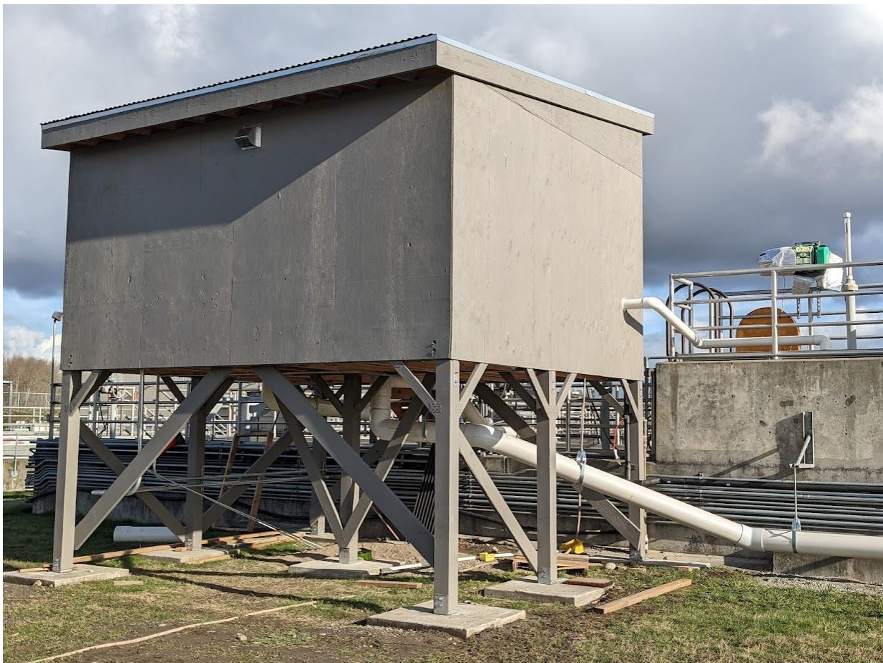
Figure 5-1. Media screen structure and temporary piping at west end of aeration basin
