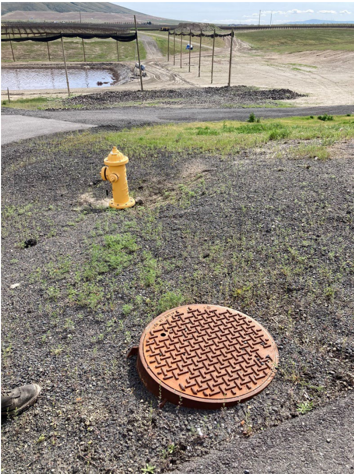
Photo 3 [IMG_0374] Description: Valve for lagoons and culvert below constructed for stormwater management
