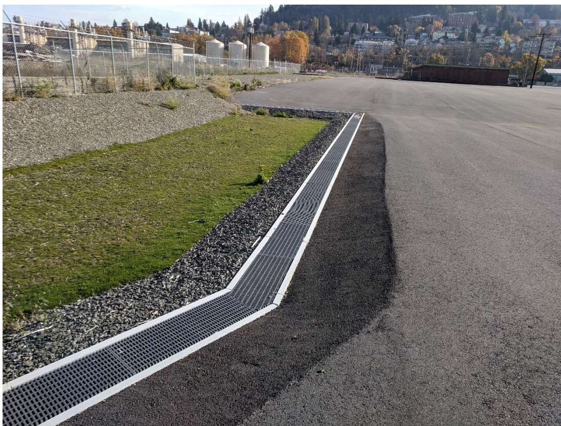
Image 3. Trench drain at the inlet to the MFD in Basin 4. Biochar filter socks would be installed either along the outside edge of the grate, or under the grate inside the concrete trough of the trench drain.
