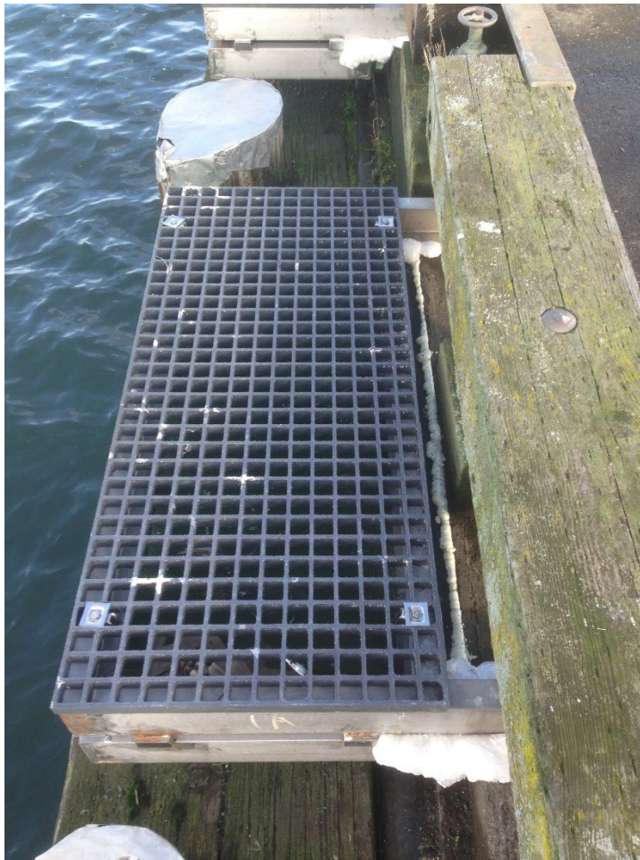
Image 2. Media filter basket installed at edge of BST Wharf.
