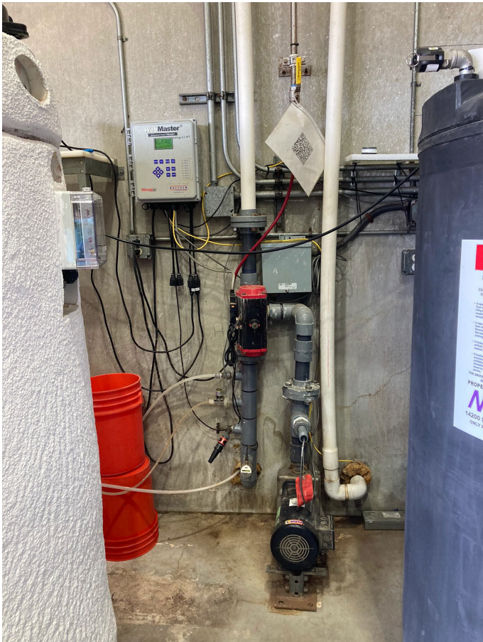
Photo 3 [IMG_0434] Description: Web Master to monitor pH, pH probe, flow meter located above – with caustic and acid dosing tanks on either side
