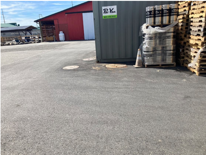
Photo 1 [IMG_0431] Description: Catch basin on the right next to the kegs and the lift station to the left of the catch basin
