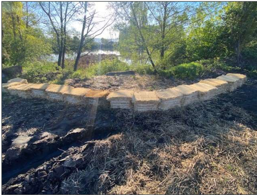
5. View of erosion control straw bales near dewatered solids pile.
