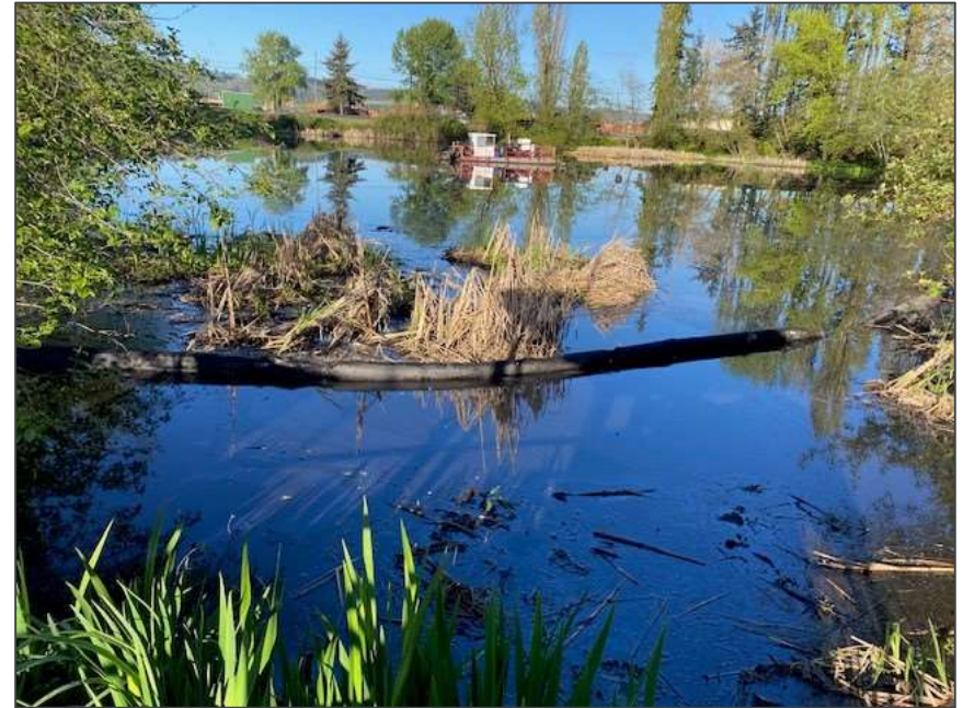
2. View of turbidity curtain in East Pond.
