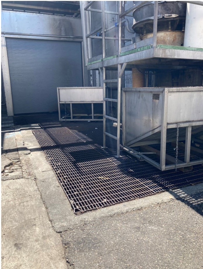
Photo 7 [IMG_0500] Description: Wastewater pit and solids bin from screening
