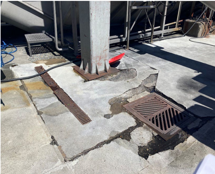
Photo 2 [IMG_0495] Description: Drains in fruit receiving area – go to wastewater pit
