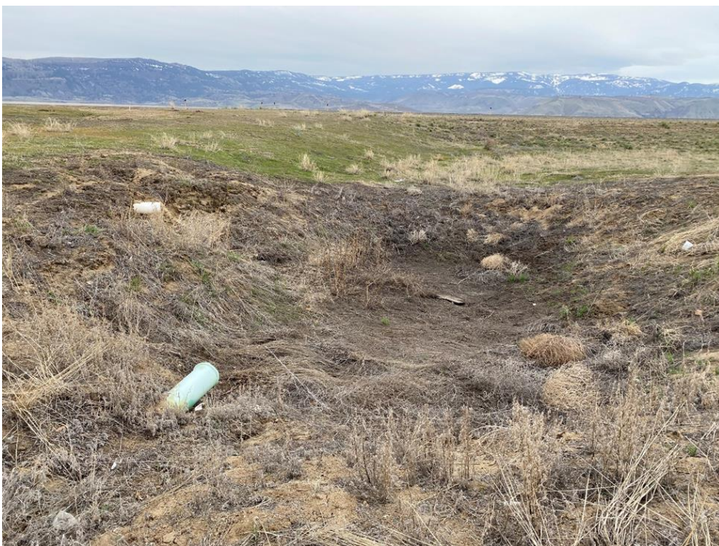
FIGURE 4. STORMWATER AND ROOF DRAIN RUNOFF INFILTRATION DEPRESSION
