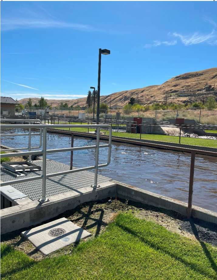
Photo 4 Description: Oxidation ditch
