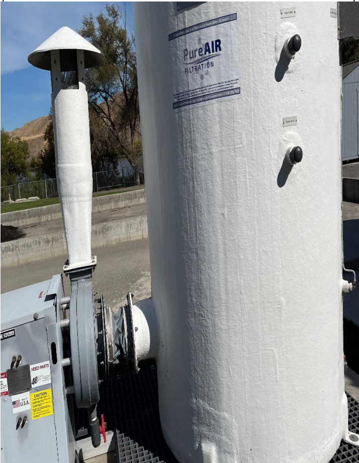
Photo 12 Description: Chlorine scrubber tank
